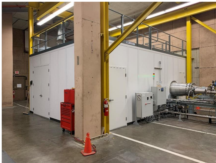
Figure 8. Test section room
