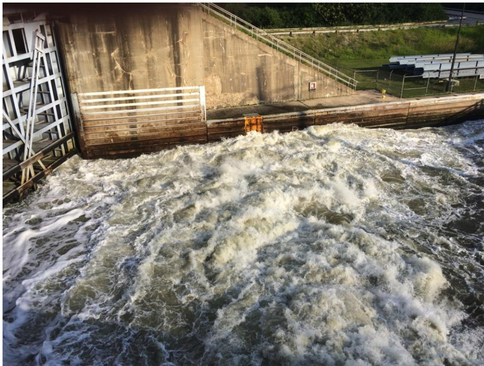
Figure 9. Turbulence in BRLD downstream approach channel during lock-chamber drain.
