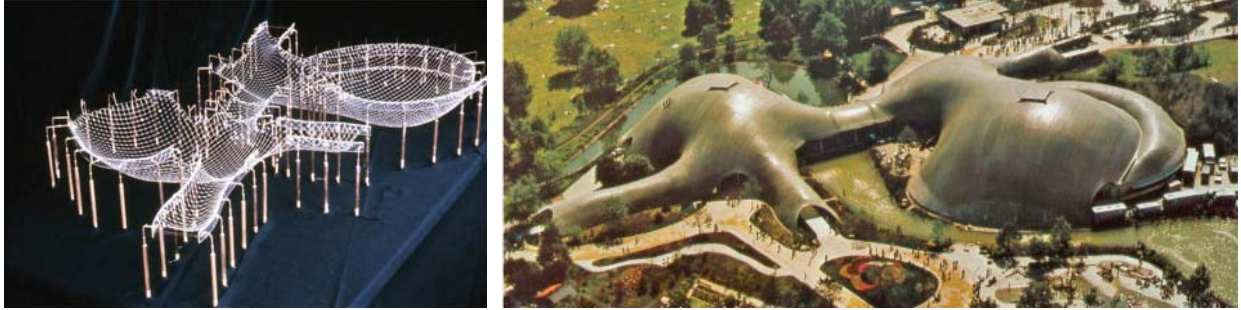
Figure 2: Mannheim Gridshell in Germany. (a) Hanging chain model [3]. (b) Constructed gridshell [4].
