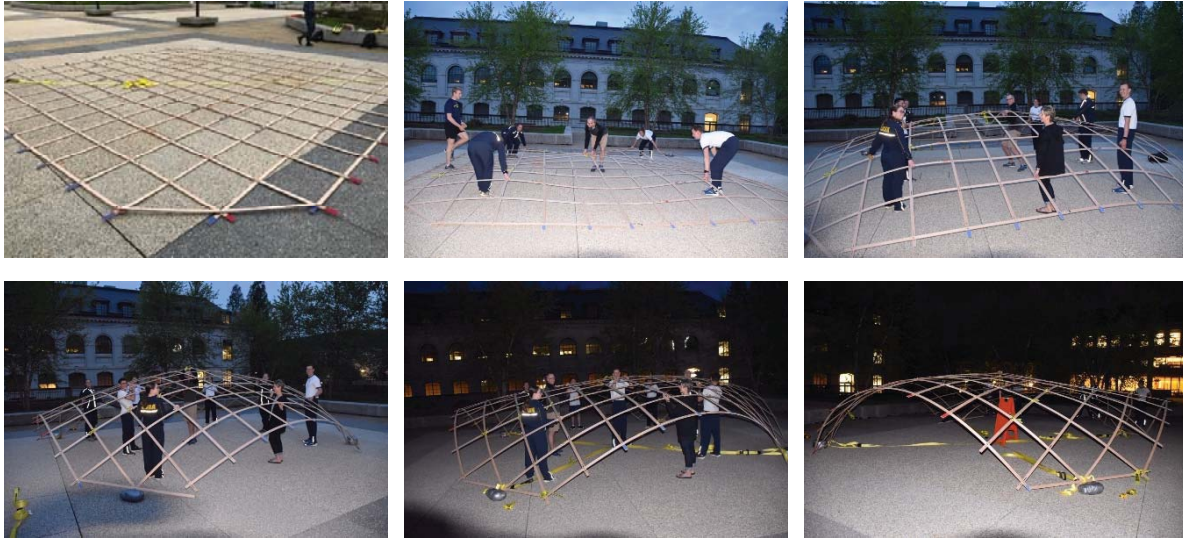
Figure 32: Construction process for prototype. (a) Lattice assembly. (b) Arch support. (c) Mid-deformation. (d) Fully deformed, weight supports in corner. (e) Tension straps added. (f) Final form achieved.
