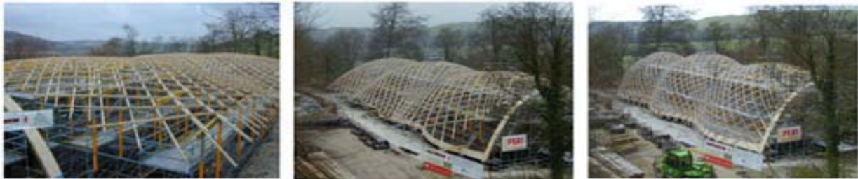
Figure 3: Time-lapse of the construction of the Downland Gridshell [2]. (a) Prior to deformation. (b) Mid-deformation. (c) Fully deformed, complete gridshell structure.
