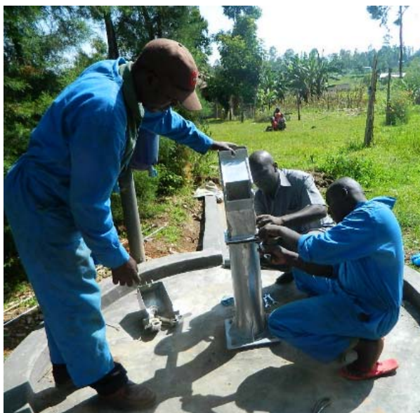
Figure 9: Kenyan community members effectively maintain and repair this hand pump that has remained functional since 2015. 156
