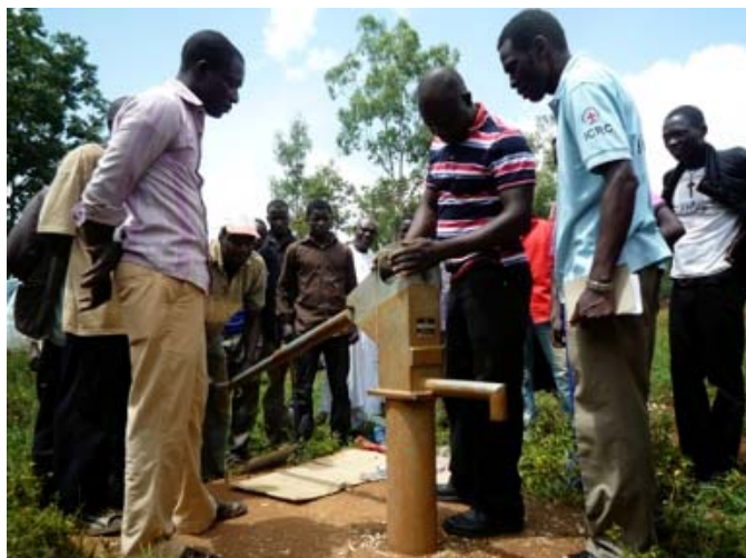
Figure 8: Nigerian community members learn to repair and maintain the pump newly installed at the Rahoss Primary School in 2012. 155
