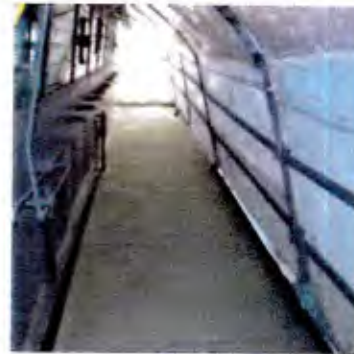
Figure 2. Example of a US Navy composite overlay installed on a ship deck. There are currently prototypes aboard 12 ships totaling 70 patches in service.
