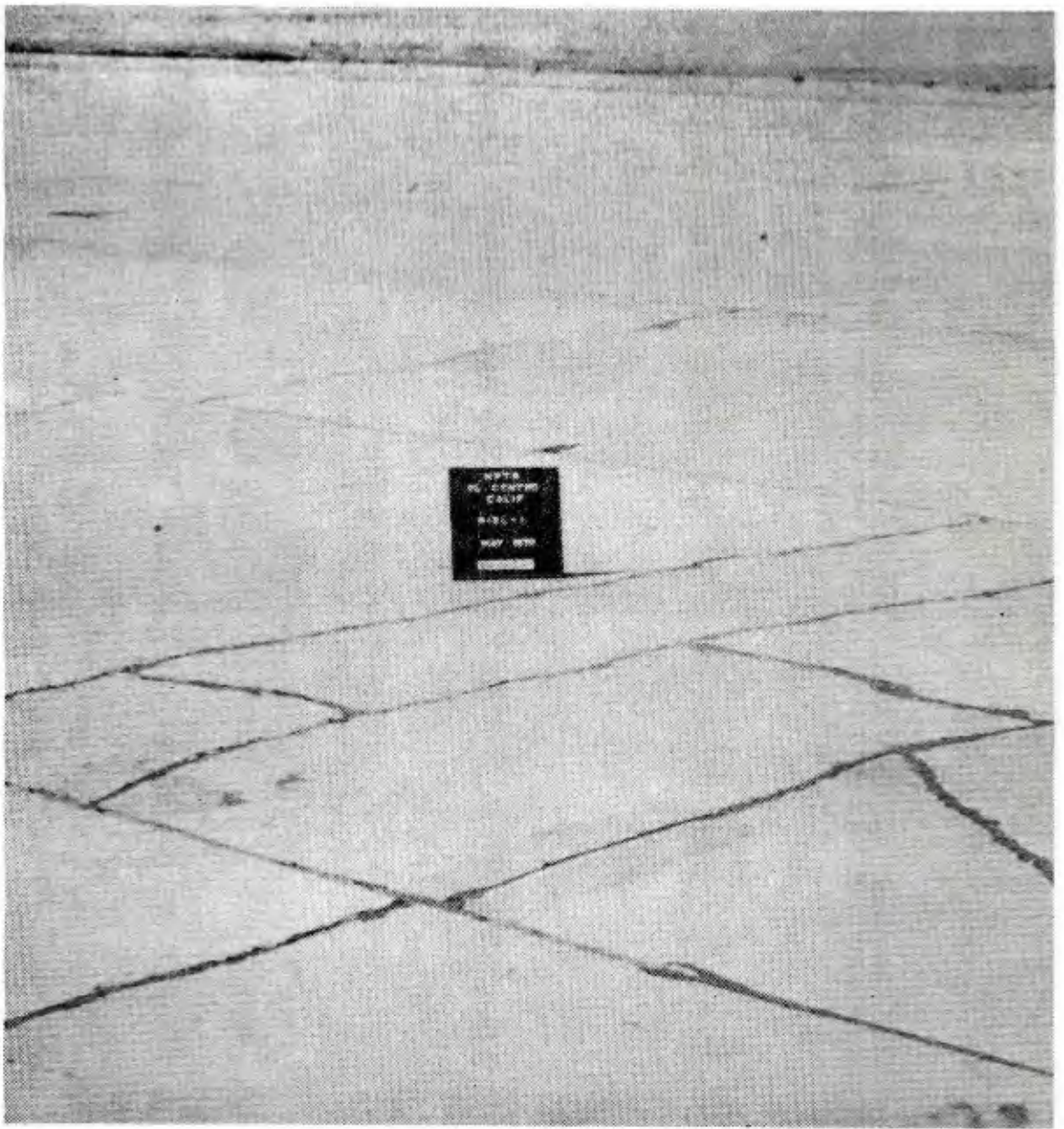
Figure 5. Shattered slab, Discrete Area R12L-1.
