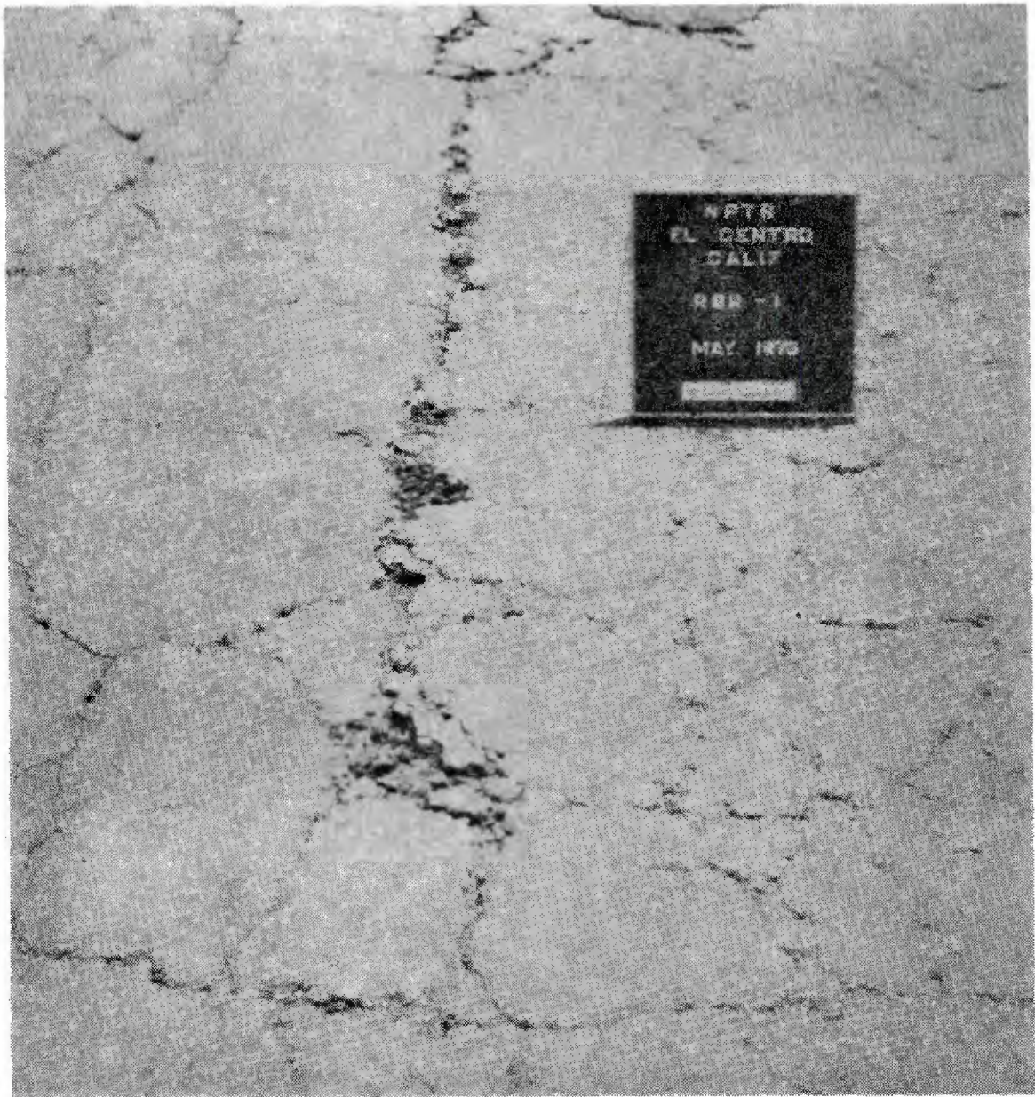
Figure 2. Severe pattern cracking and raveling, Discrete Area R8R-1.
