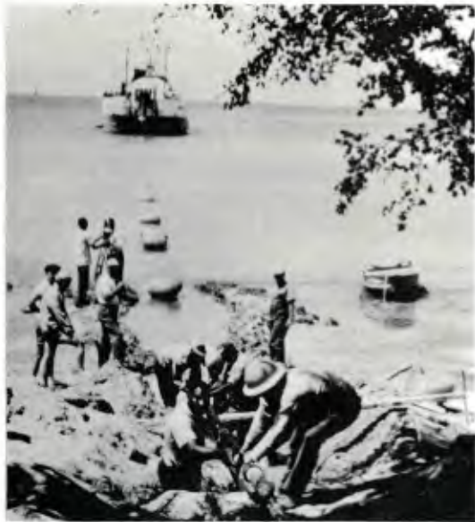
Figure B-1. Trenching the Shore End
