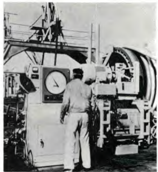
Figure B-4. Tensioning Control Console and Capstan
