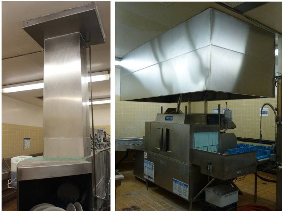
Figure 26. Baseline and Demonstration Ventilation System
