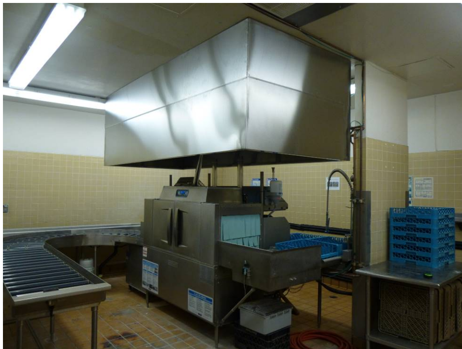
Figure 9. Demonstration Dish Room Layout
