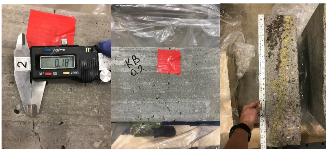
Figure 40. Kwik Bond Slab Specimen at 0.2 mm
