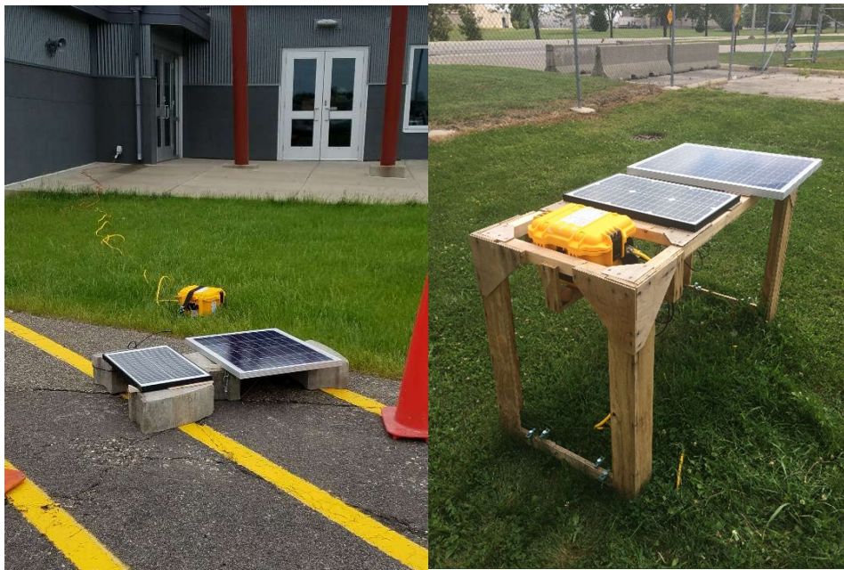
Figure 13: Grid connected test systems, St. Paul Air National Guard Base, MN (Left) and Grissom Air Reserve Base, IN (Right)
