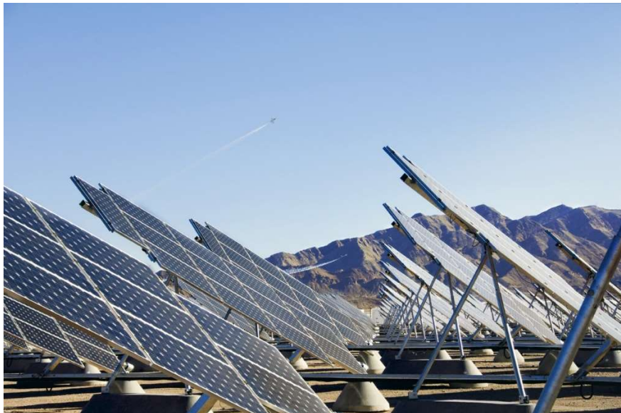
Figure 2: Second solar array constructed at Nellis, AFB [17]
