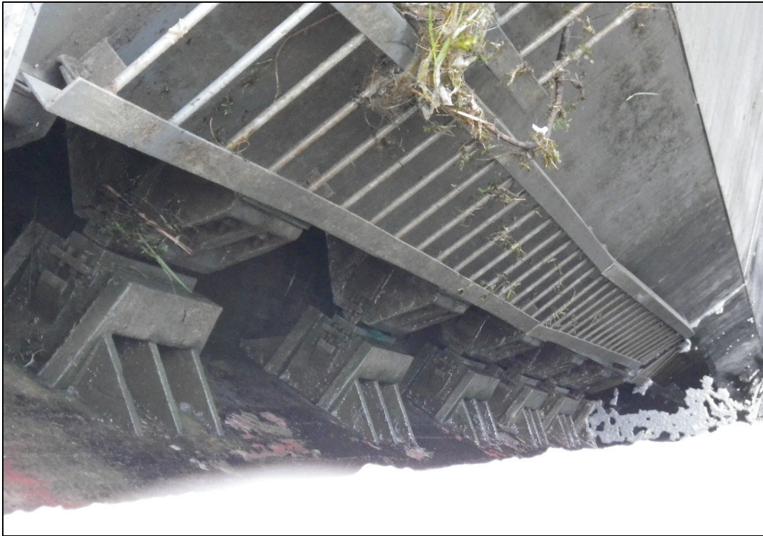
Figure 12. Locks on the Dnieper River, Ukraine, showing intermittent contact surfaces.
