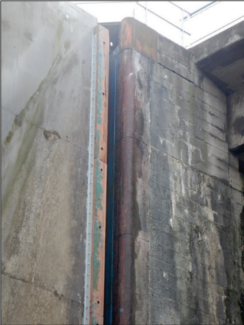
Figure 13. Supplementary water seal at Diepenbeek lock.
