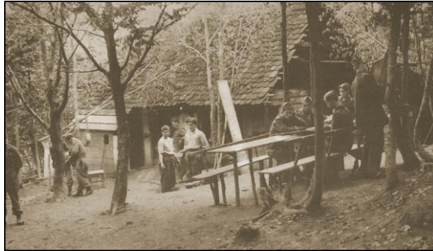
Figure 2: Central Partisan Hospital on Petrova Gora, 1944 14
