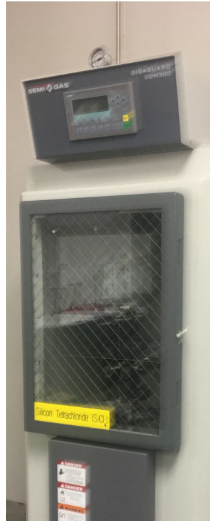
Fig. 7. Picture of the installed liquid push system for Silicon Tetrachloride and Germanium Tetrachloride.
