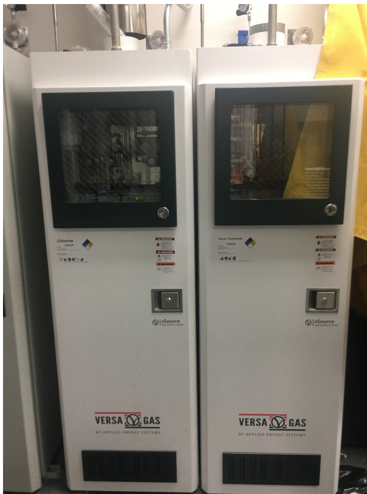
Fig. 5. Gas cabinets for \text{Cl}_2 and \text{BCl}_3 gases have been purchased from AES.
