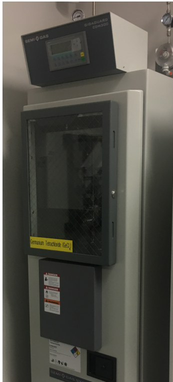
Fig. 7. Picture of the installed liquid push system for Silicon Tetrachloride and Germanium Tetrachloride.
