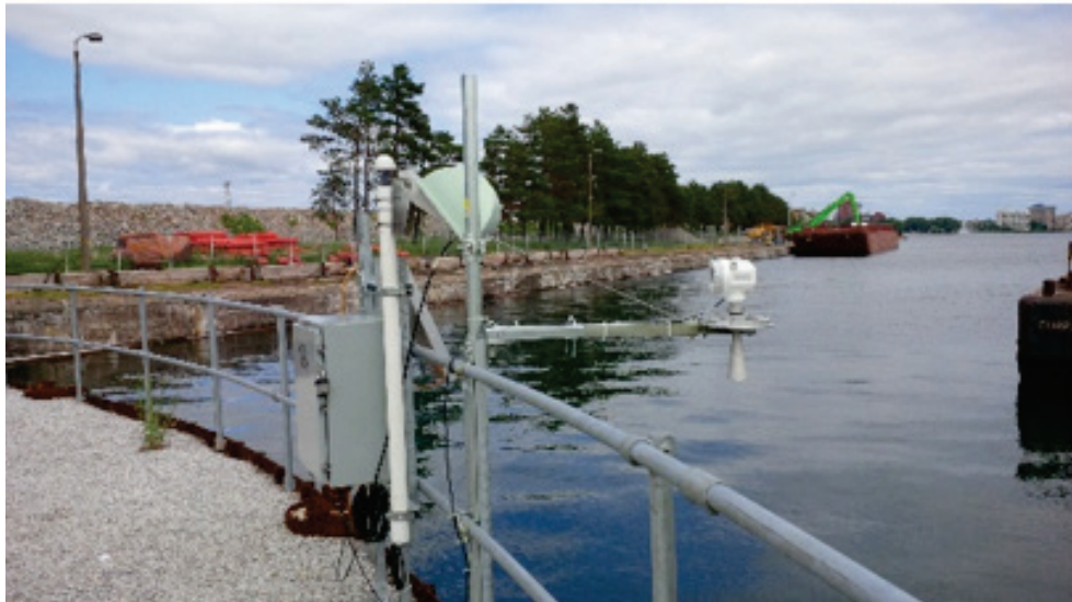
Figure 7. Downstream radar gauge placed on a coffer dam.
