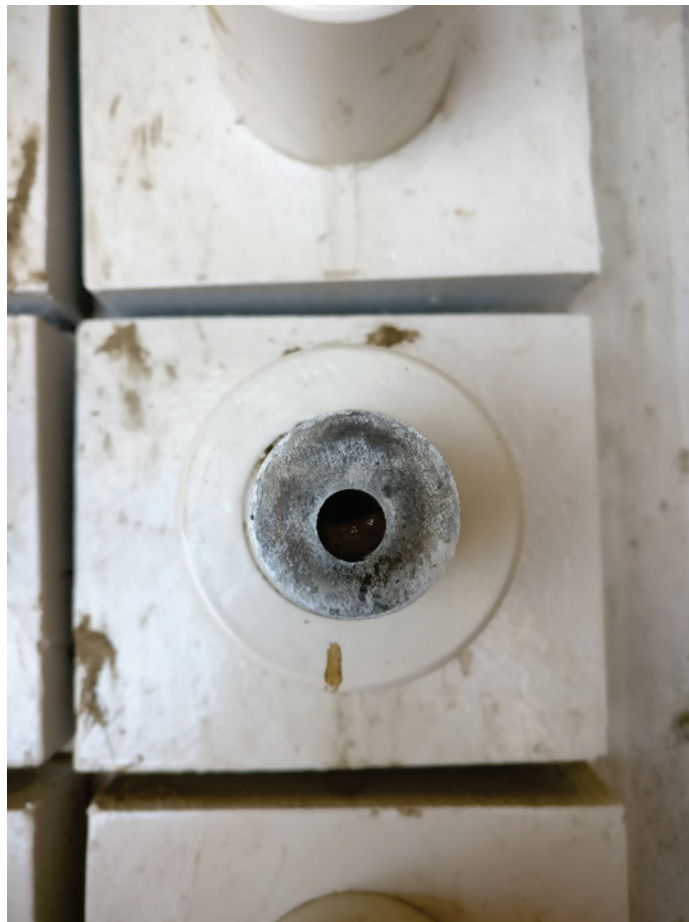
Figure 2. Drilled tendon at Oroville Dam.
