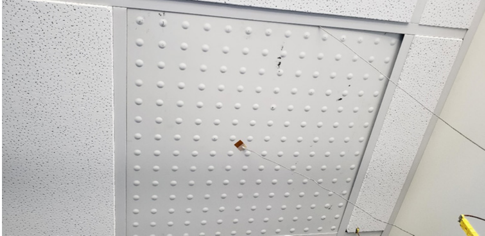
Figure 8. PCM panel placed in the ceiling
