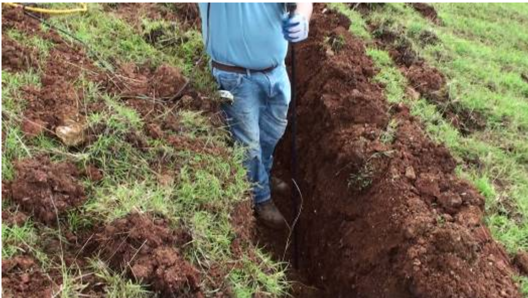
Figure A4. Cathode rod being driven into the ground.
