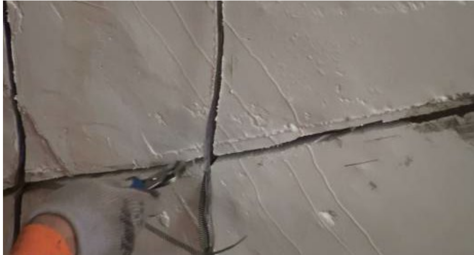
Figure A9. Ceiling anodes.
