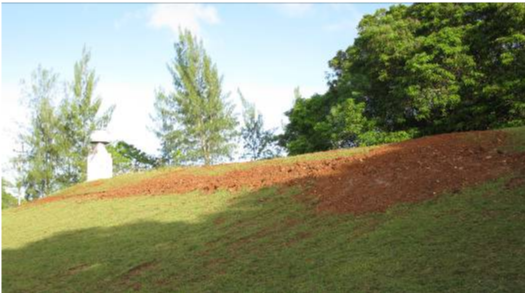
Figure A12. Cathode trench backfilled.
