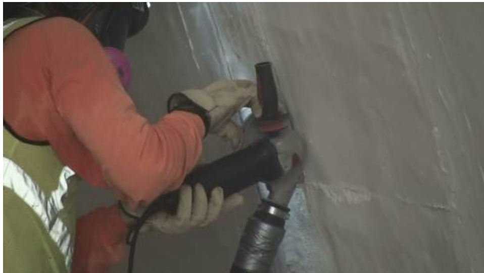
Figure A5. Ceiling cut for anode installation.
