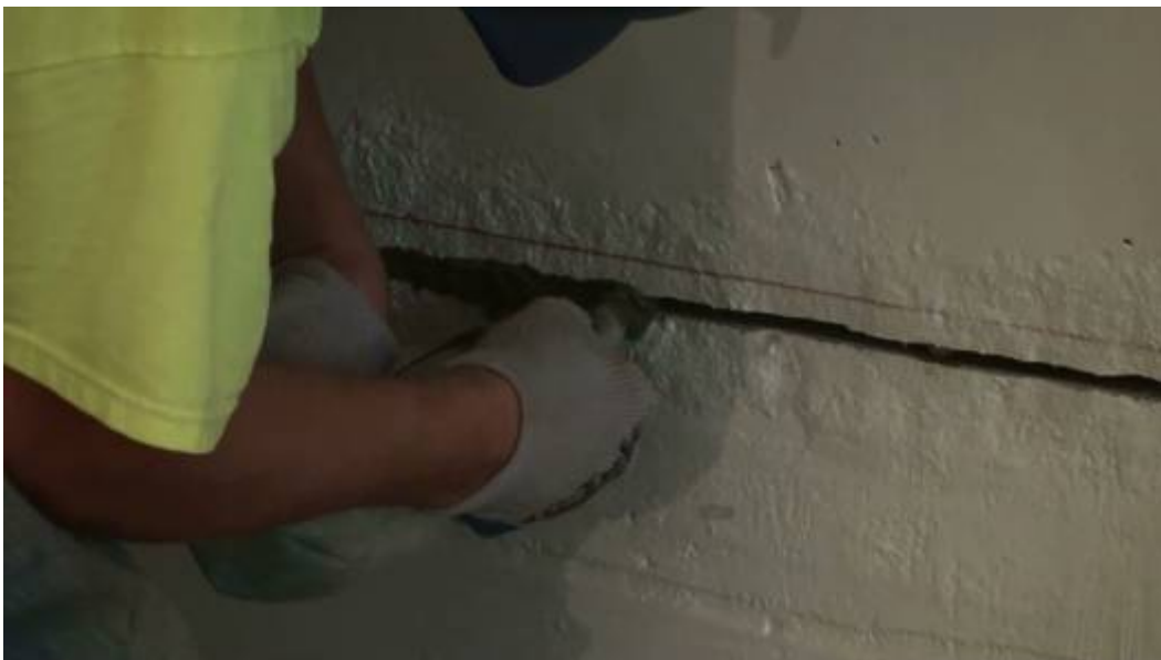
Figure A10. Grouting groove with cement.
