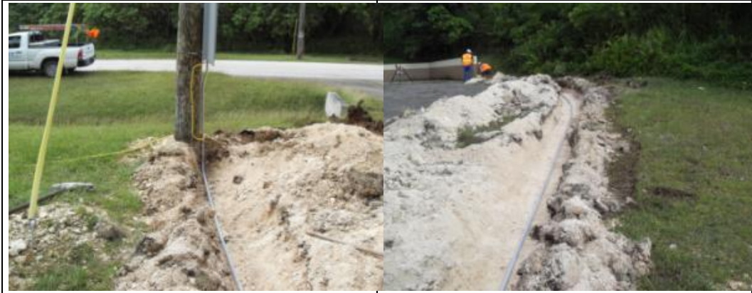
Figure C7. Installation of buried electrical line for Guam ECM 12AC20.
