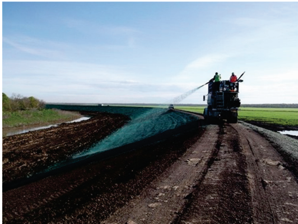
Figure 7. Addition of hydromulch, grass seed and biopolymer to soil on Kaufman Levee, spring, 2014.
