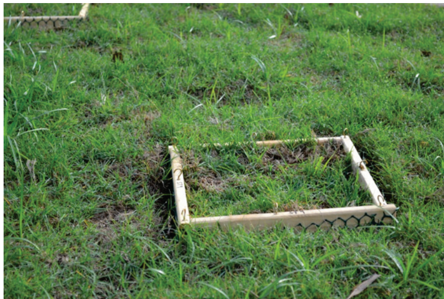
Figure 4. Pull box designed and placed in the field under sod.
