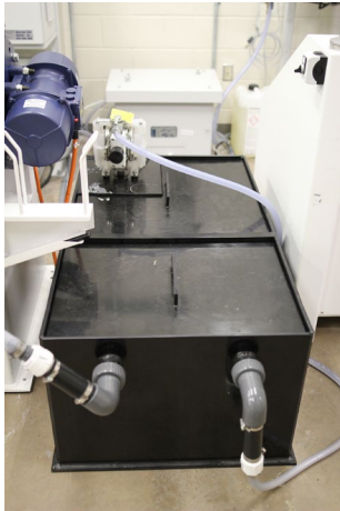
Figure 5. AB04 Weir Tank
