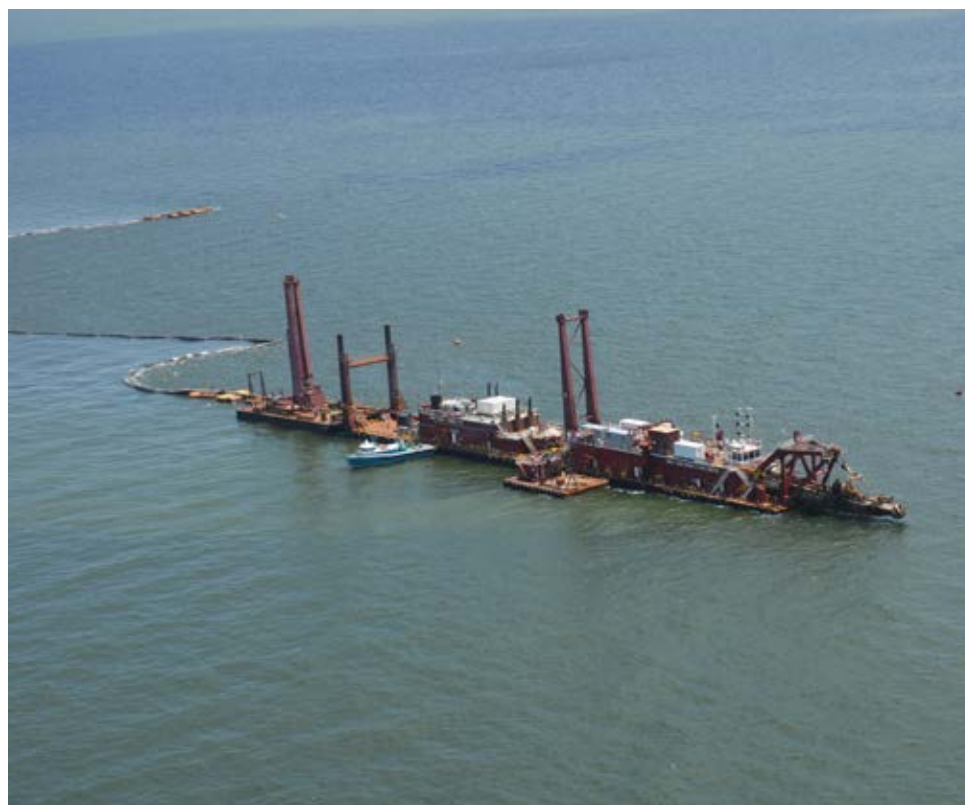
Top: Pipe used for pumping sediment from hydraulic cutter-head dredge to placement area. Sand berms were constructed along sensitive barrier islands to reduce impacts from the Deepwater Horizon oil spill. (Photo by Louisiana Coastal Protection and Restoration Authority)
