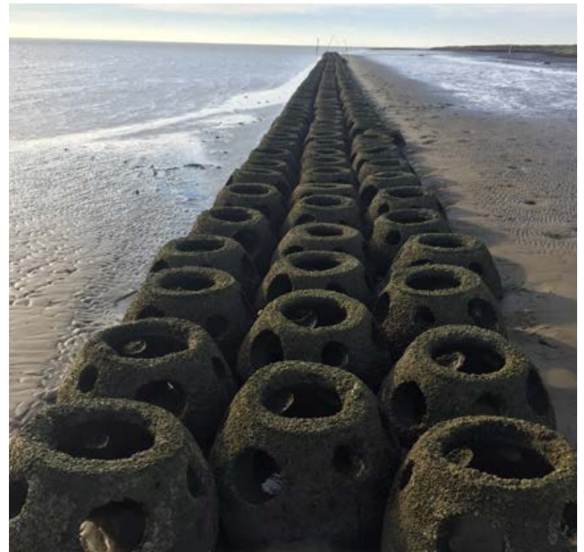
Bottom: Reef Balls form a breakwater. (Photo by Mary Kate Brown, The Nature Conservancy)
