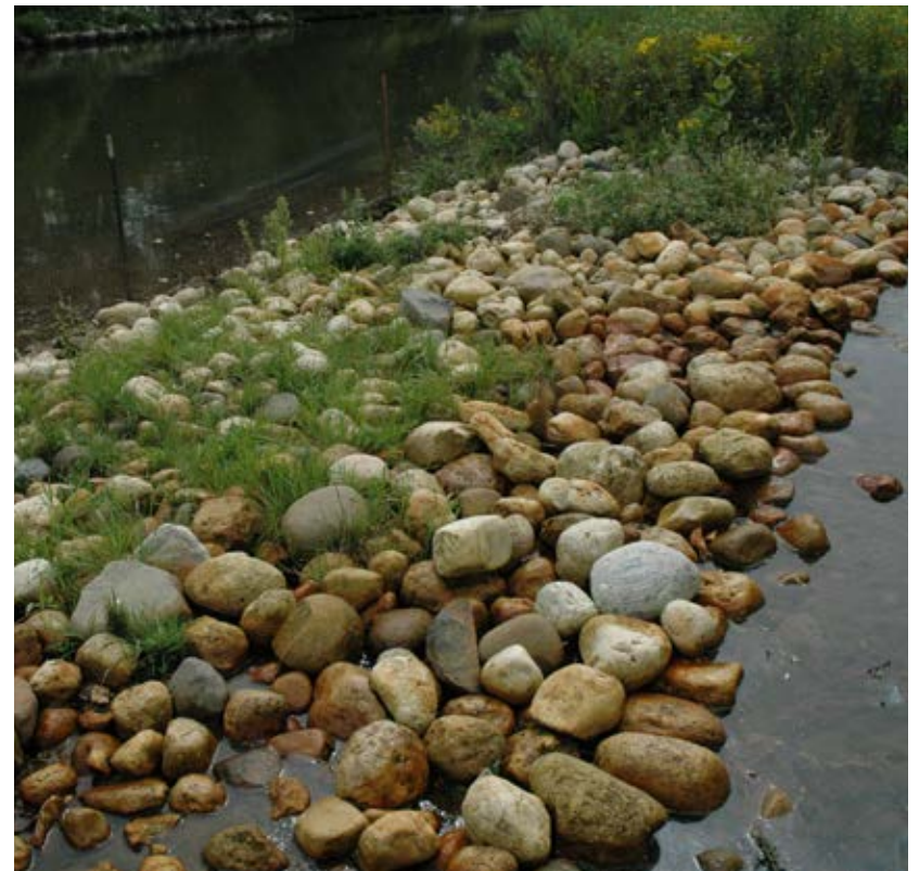
Bottom: Cobble bars help prevent erosion and stabilize the banks. (Photo by USACE Chicago District)
