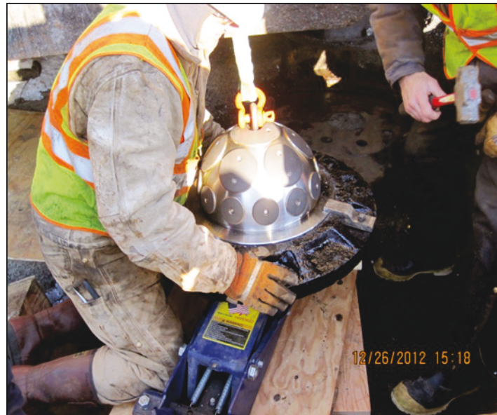
Figure 14. A self-lubricating pintle bearing.
