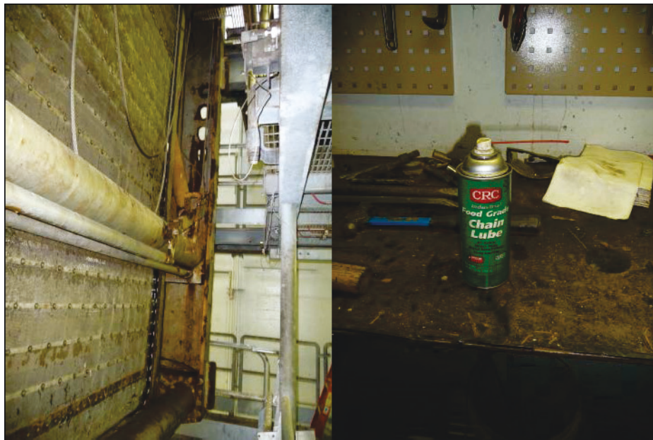
Figure 11. Left- Fish screen undergoing maintenance at John Day Dam, OR. Right- Spray-on chain lubricant.
