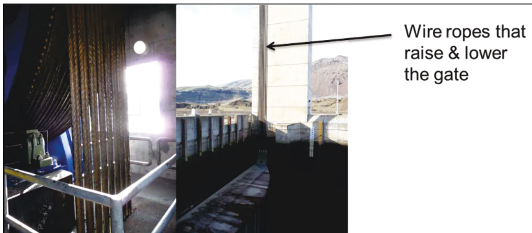
Figure 17. The downstream gate at John Day Dam. A rotating drum raises and lowers the gate via heavily greased wire ropes.
