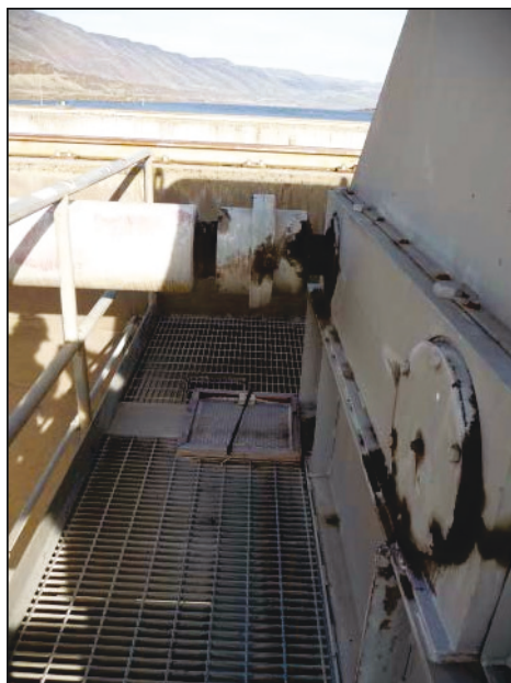
Figure 24. Suspended gate motor showing lubricant leakage at The Dalles. Sorbent pads controlled dripping below.
