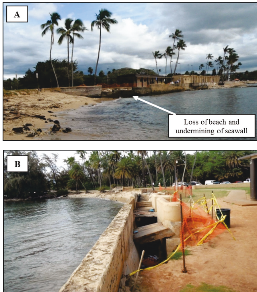
Figure 3. Pictures from the March 2017 site visit showing the severe erosion of the beach at the northern section of the Haleiwa Beach Project (A) and the washed out area behind the seawall (B).
