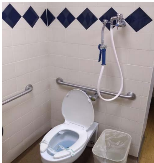
Figure 1: Bedpan Washing Toilet Station at University of Oklahoma Medical Center
