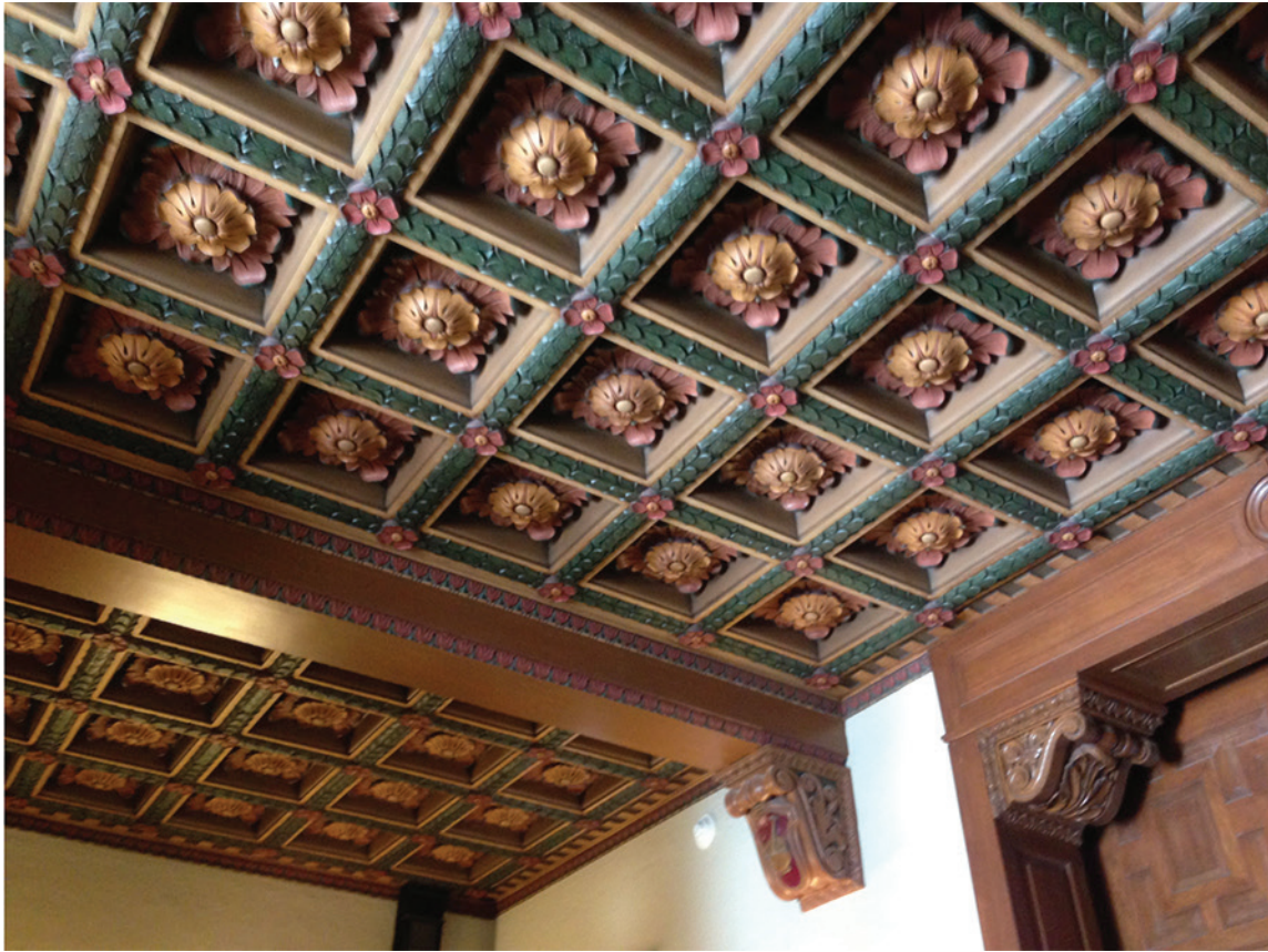
Figure A.3 Ceiling of the Foyer in the BAMC Building
