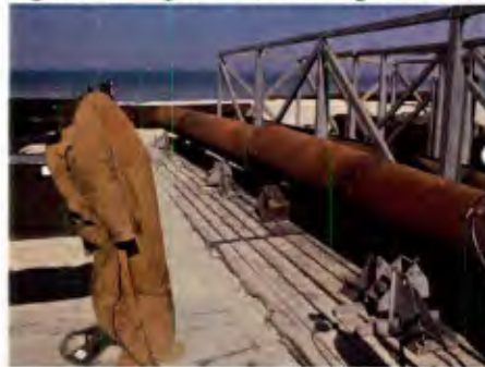
Rapid Pile Splicer (existing rollers)
