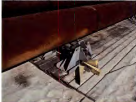
Rapid Pile Splicer (existing rollers)
