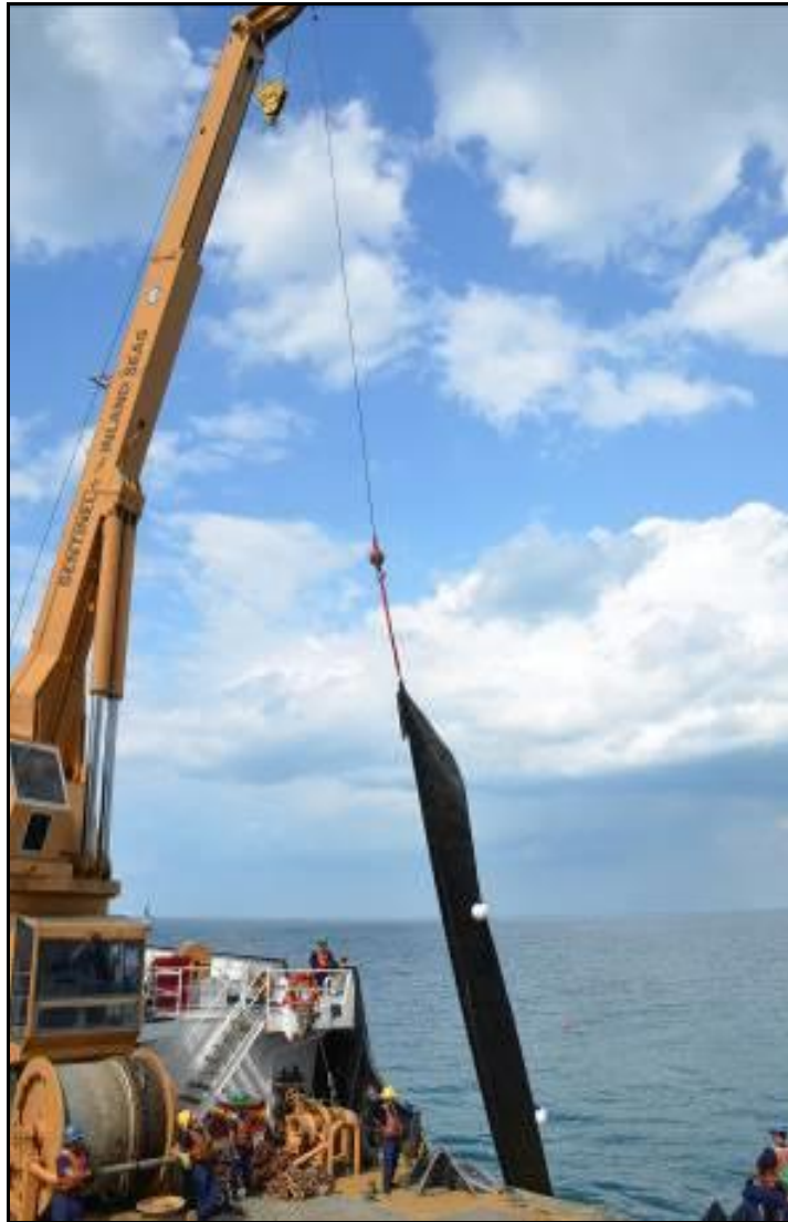
Figure 44. Attempt to recover the offshore mitigation system with crane during high-wind conditions.
