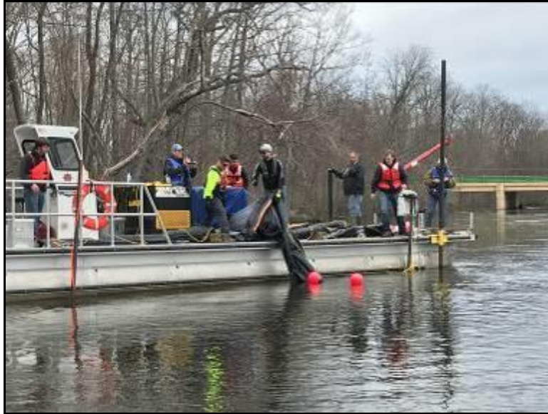
Figure 21. Inland mitigation system 1 prototype being deployed using the anchor post method.
