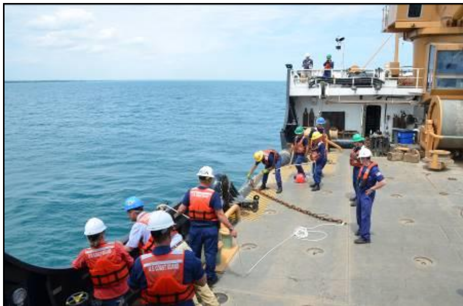
Figure 39. Second and final anchor dropped into Lake Huron after positioning system into an U-shape configuration.
