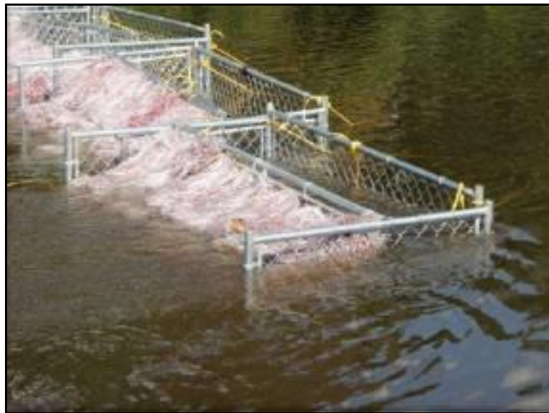
Figure 1. Gabion basket with snare booms in the Kalamazoo River during 2012 cleanup efforts (Enbridge Energy, 2016).
