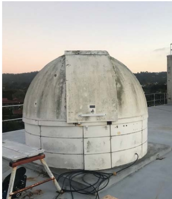
Figure 26. Existing Telescope Dome at NPS
