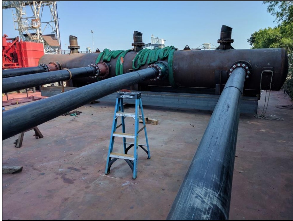
Figure 3-2. Jet manifold awaiting deployment in the CSSC. The photograph shows the 0.3 m diameter fused HDP pipe connected to the four 0.41 m side ports through a reducer. The three 0.3 m jet nozzles are visible on the top of the manifold. Steel bridge piers were mounted on the manifold feet to provide anchor support. One is visible beneath the side ports. When placed in the canal, the jets are oriented upstream.
