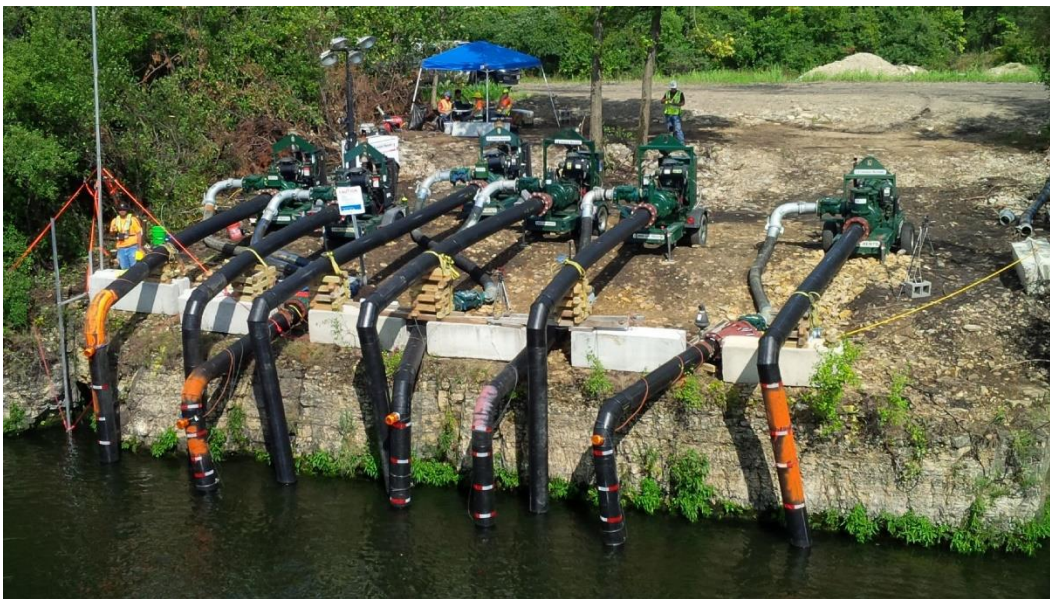
Figure 3-5. East bank operations area depicting the pump setup. There are six intake lines and four discharge lines that supply water pressure to the jets. The six intakes are set on top of the Jersey barriers and supported by the wooden slats. The four discharge pipes are set between the Jersey barriers. The strobe lights are visible on four of the pipes. A light plant (top, center, left) was also deployed to illuminate the site at night.
