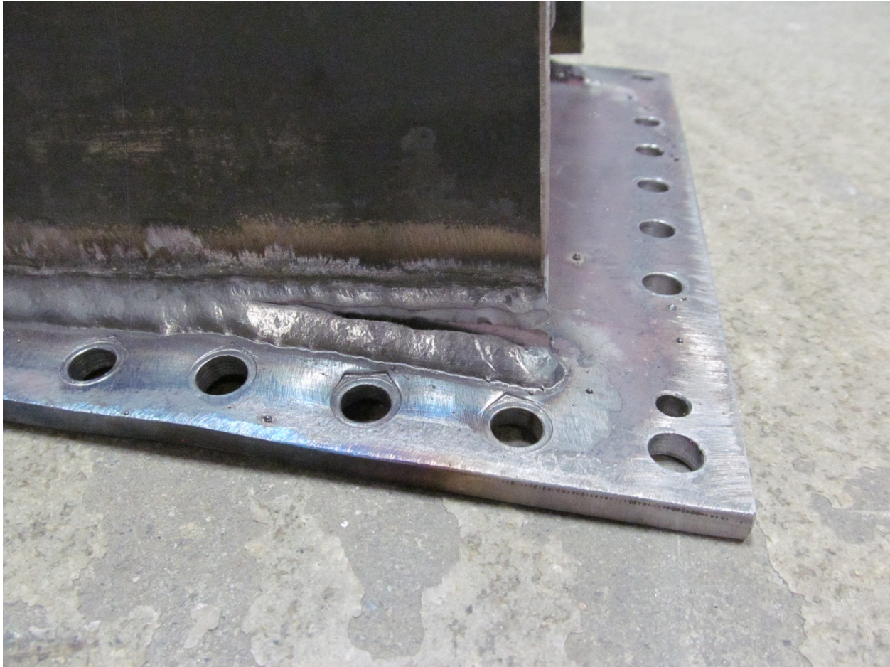
Figure 22. Crack at Position 2 on TC15
