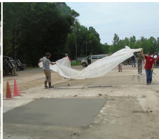
(f) Covering test section with plastic
