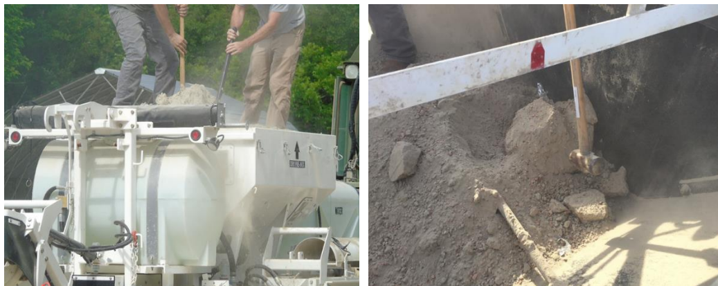
Figure 27. Large portions of compacted MPC material being broken down.
