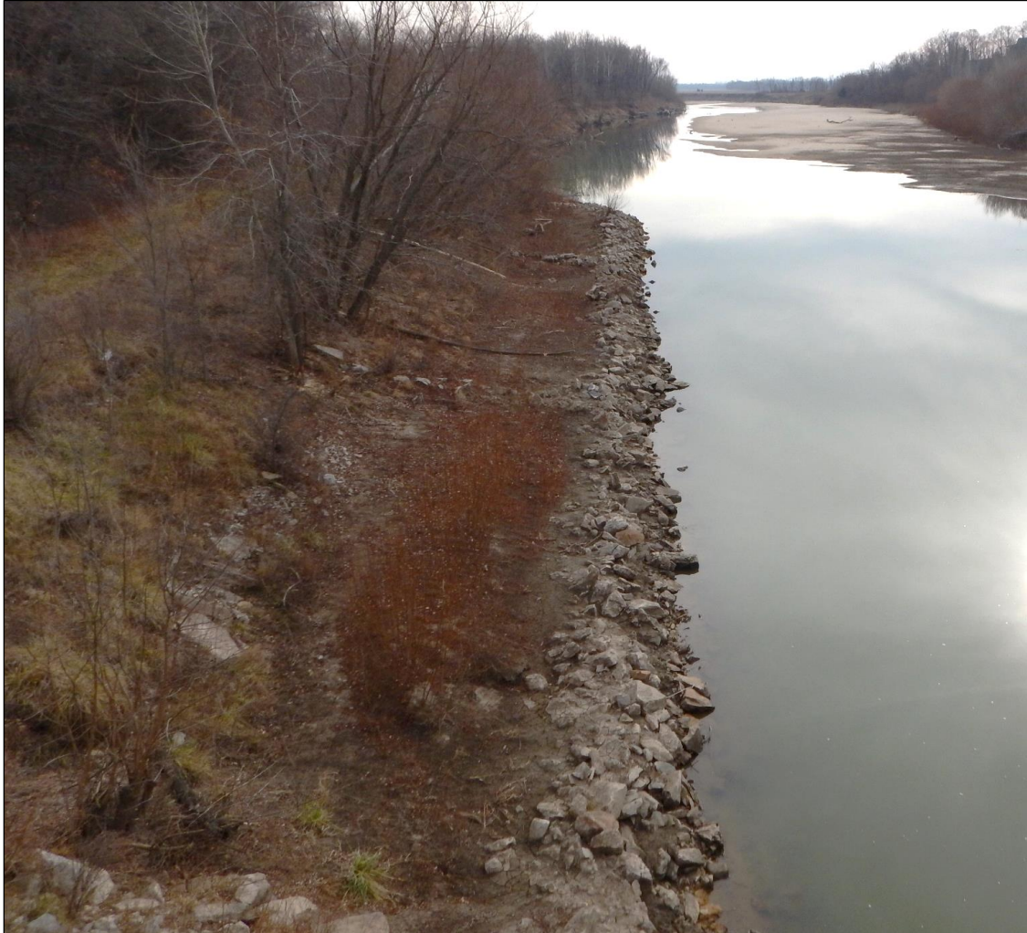
Figure 10. Successful baffle dike with longitudinal peaked stone toe protection and tiebacks at Highway 6 Section 14 project. Note significant sediment deposition between dikes.
