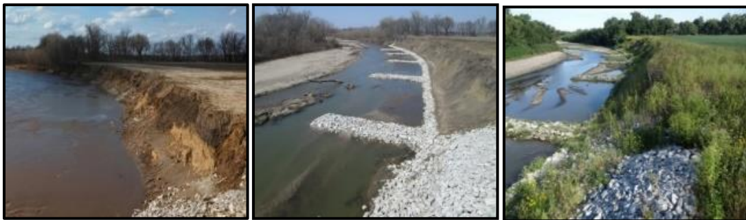
Figure 11. Successful bendway weirs with toe protection – Initial condition (left photo), after construction (middle photo), current condition Highway N (right photo).
