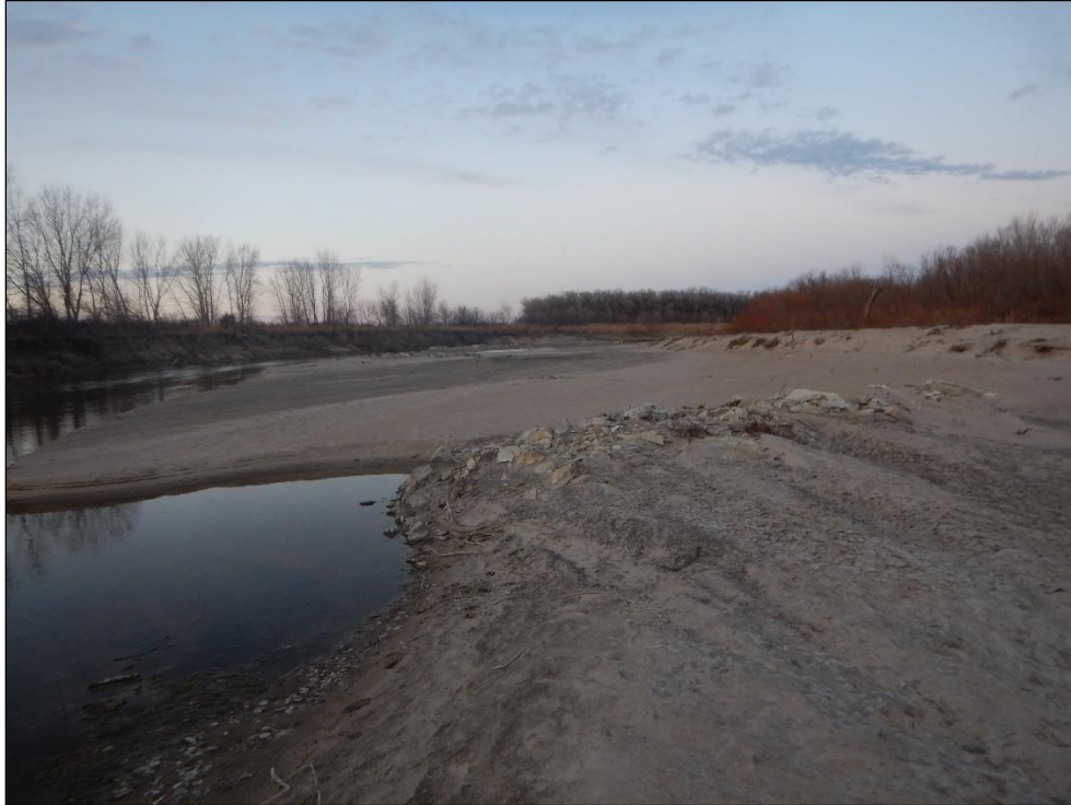
Figure 7. RR1 failure – Flanked structure buried in point bar.
