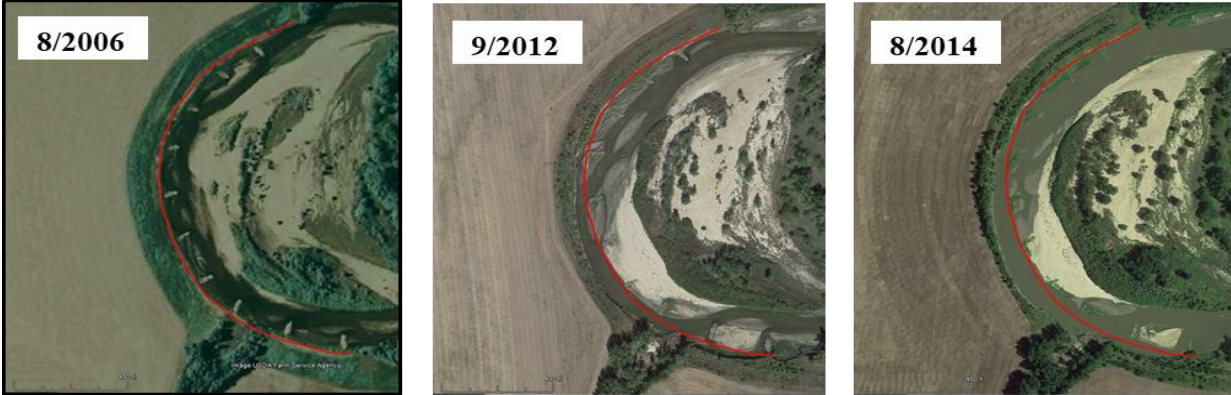
Figure 6. RR3 project site – Post construction (8/2006), After failure (9/2012) and (8/2014). (Red line indicates location of 2006 bank)
