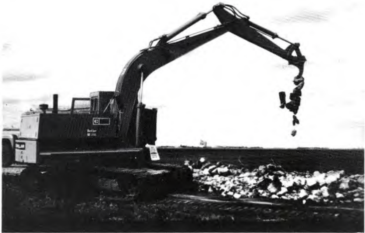
FIGURE 6. STEEL REMOVAL OPERATION USING A "RHINO HORN."
