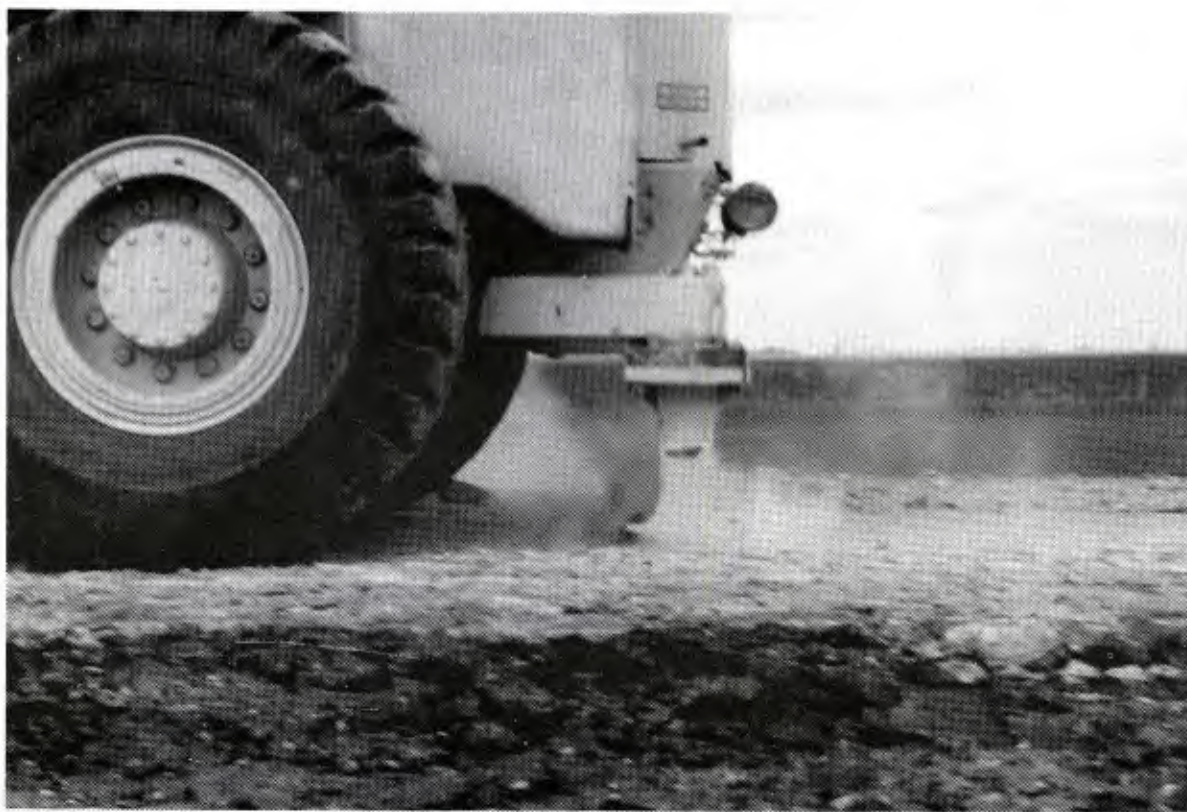
FIGURE 3. CLOSEUP OF THE IMPACT HEAD OF THE VIBRATING BEAM PAVEMENT BREAKER.
