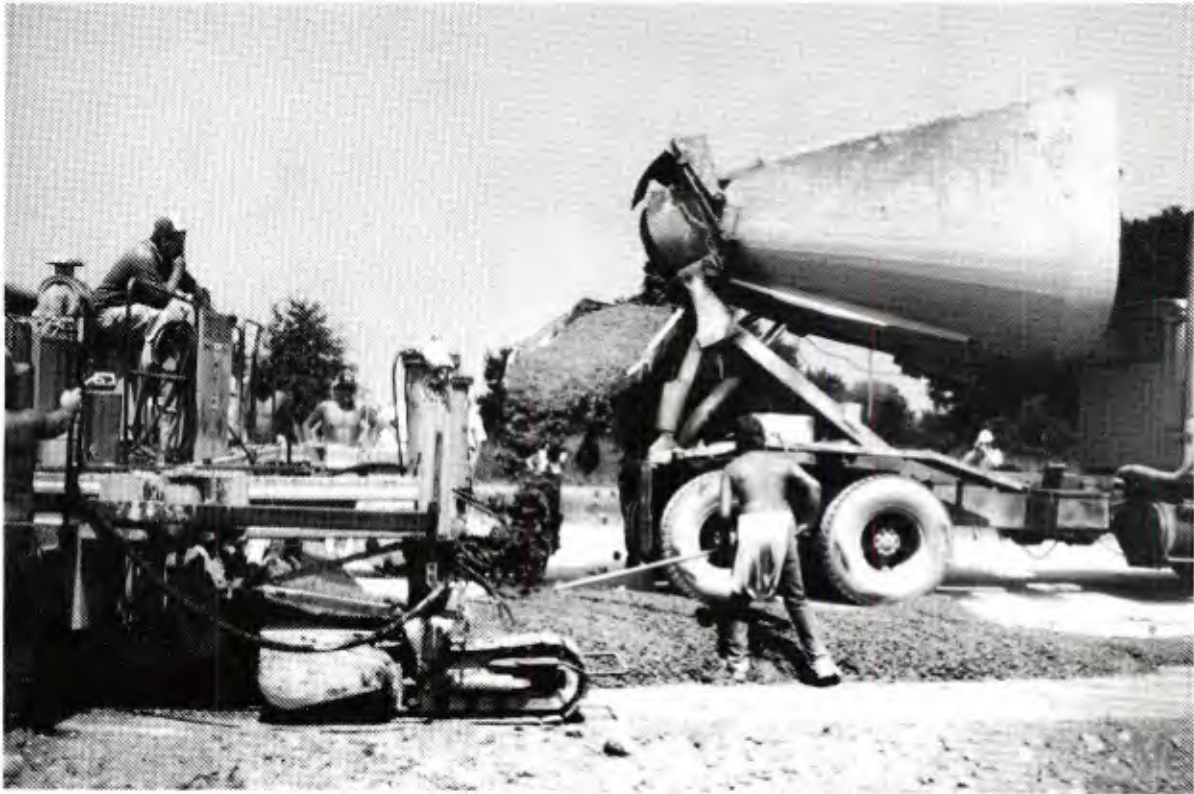
FIGURE 8. PAVING RECYCLED PCC MIX WITH CONVENTIONAL EQUIPMENT AND PROCEDURES (Interstate 94, west of Battle Creek, Michigan).
