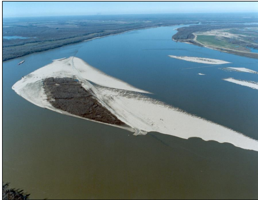
Figure 122. Looking upstream at Smithland Crossing after construction of dikes. The chute closure structure has not been completed, the river has not eroded to the trench fill revetment, and sediment has begun to deposit in the dike field.
