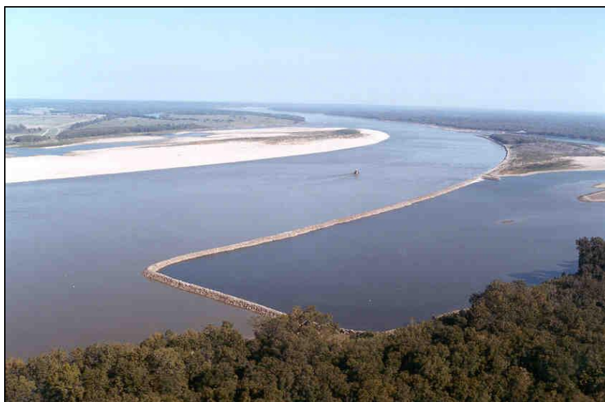
Figure 123. Smithland Crossing after completion of chute closure structure. Looking downstream — the river has eroded back to the trench fill revetment, and sediment has deposited in dike field.
