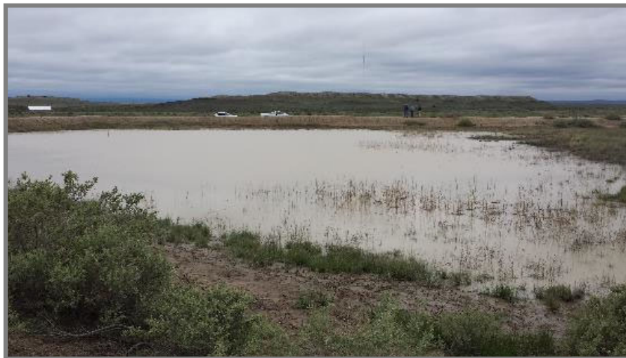
Figure 6. Erosion control dam at PCMS
