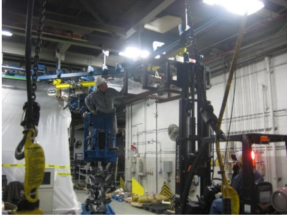
Figure 6: Overhead Trolley Removal
