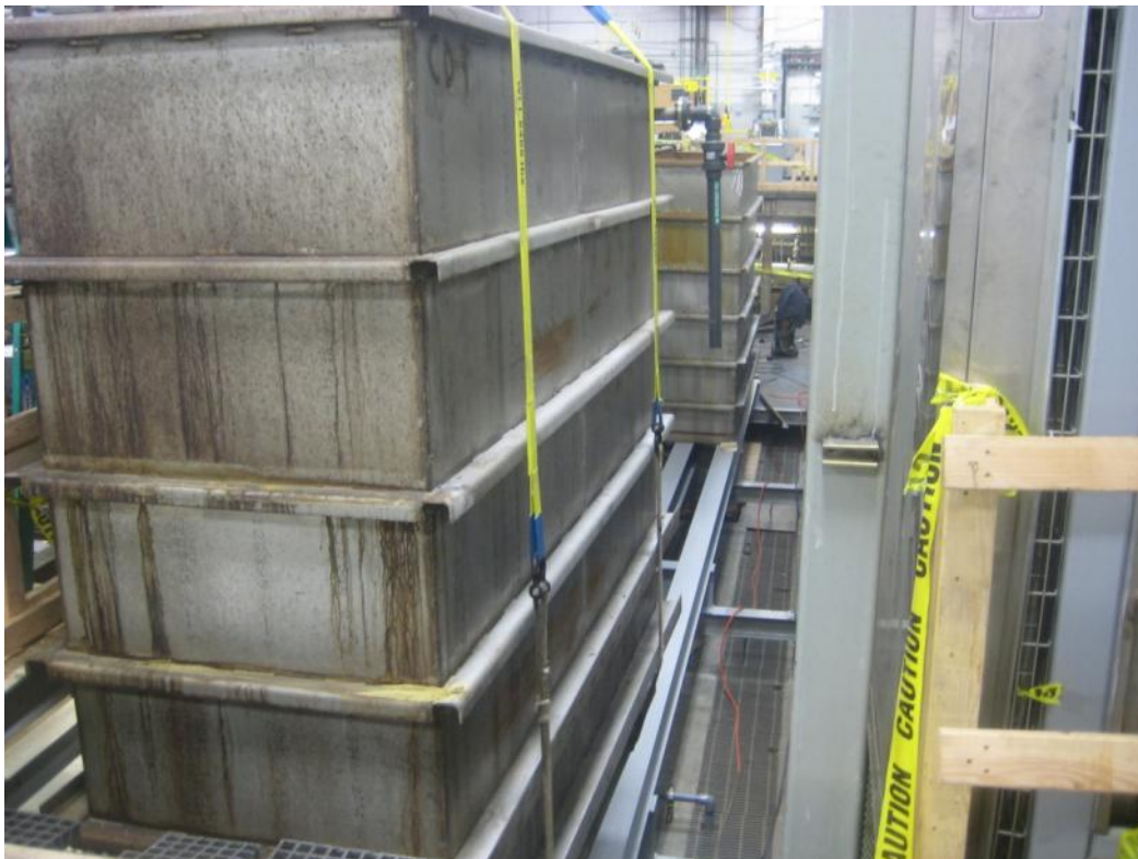
Figure 9: Iridite Tank Line Relocation
