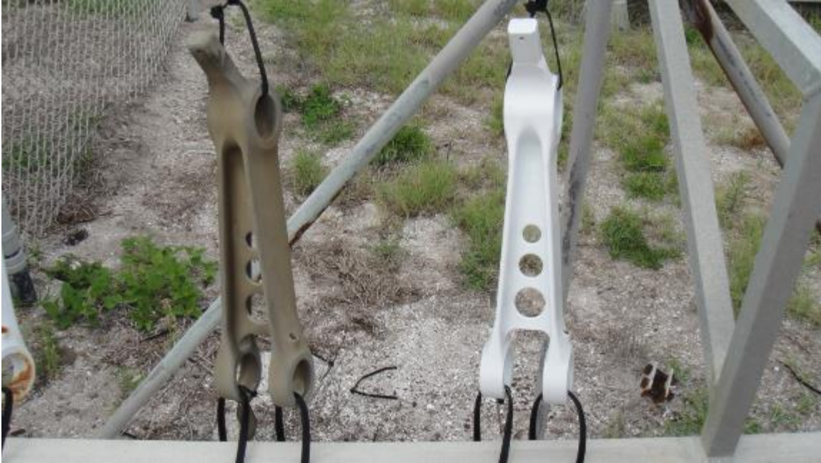
Figure 116: Cd Plated Drag Braces (8/26/2016)
