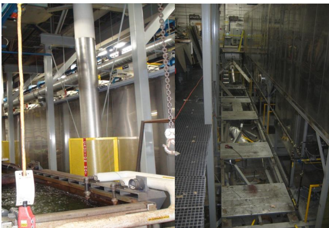
Figure 5: Industrial Oven Removal
