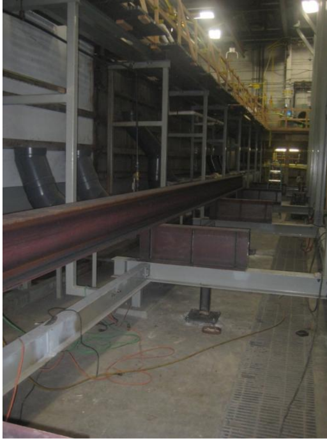
Figure 7: Footing and Structure Re-Establishment
