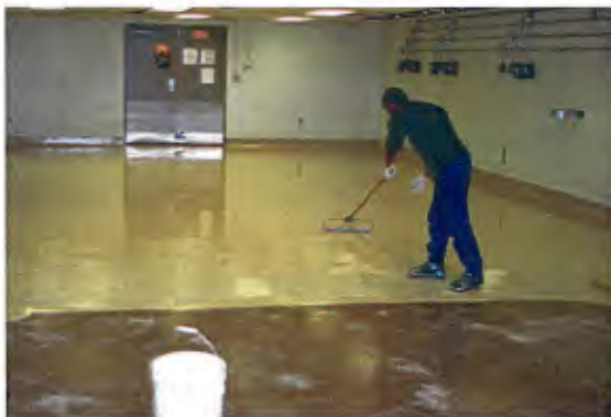
Application of topcoat.
