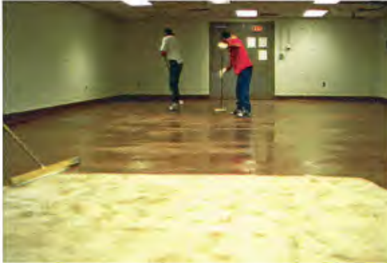
Application of grout coat.
