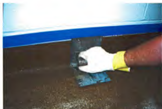
Cove trowel used to finish vertical walls.
