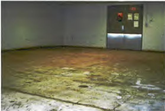
Resulting surface following degreasing.
