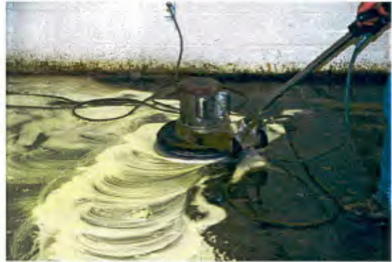
Tile adhesive removal using mechanical scrubbing and organic solvents.
