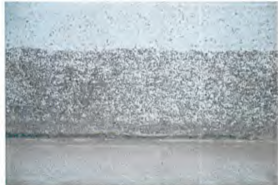
Resulting CMU profile from grinding (ICRI CSP 2).
