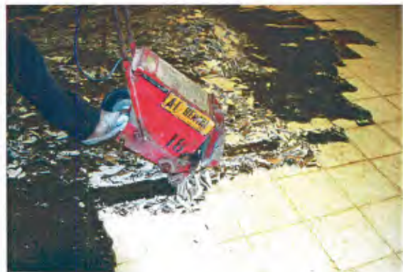
Power tool chipping.
