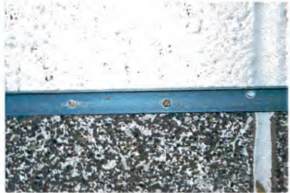
Cove strip installed for aesthetics.
