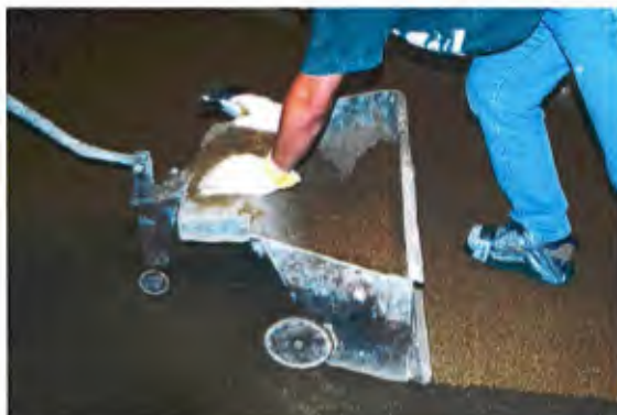
Screed application of intermediate coat.
