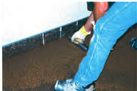
Trowel application of intermediate coat.
