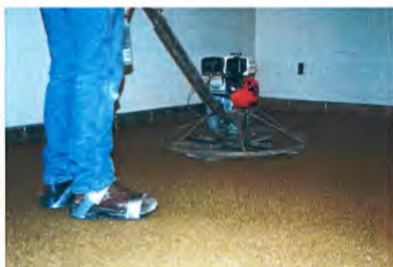
Power trowel used to finish intermediate coat.
