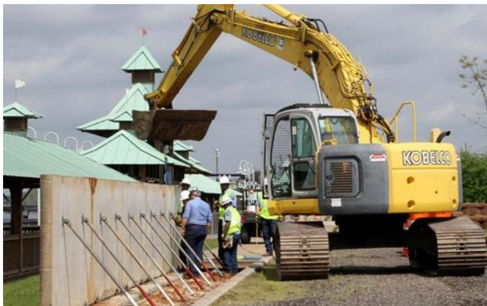
Figure 5. Monroe Solution floodwall being put in place.
