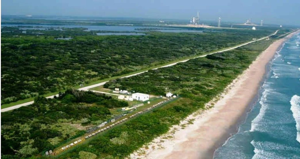
Fig. 2 NASA beachside corrosion test site
