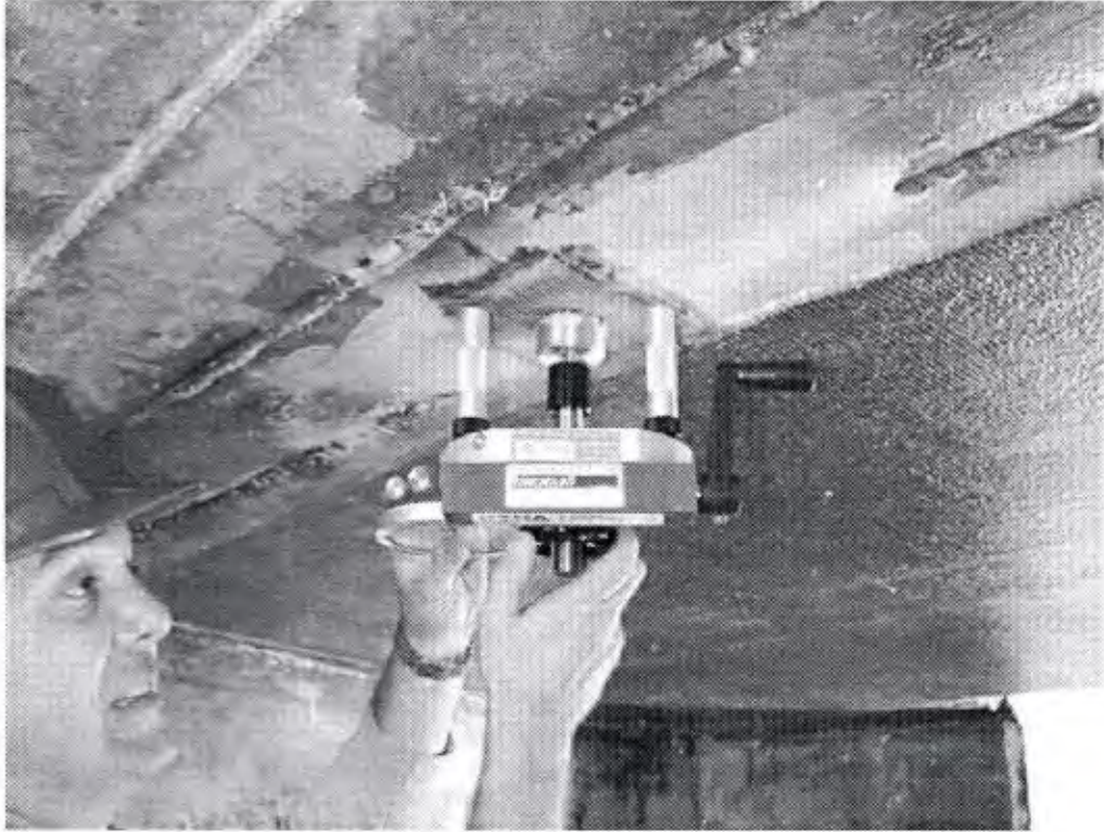
Figure 27. Bond testing with pull-off tester.
