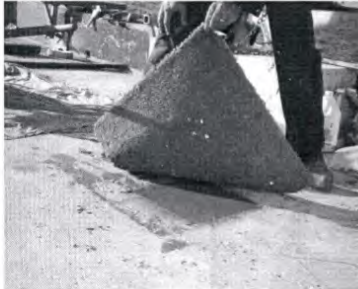
Figure 26. Wet curing concrete repair area.
