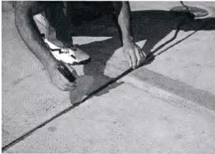
Figure 20. Installing backer rod to seal crack.
