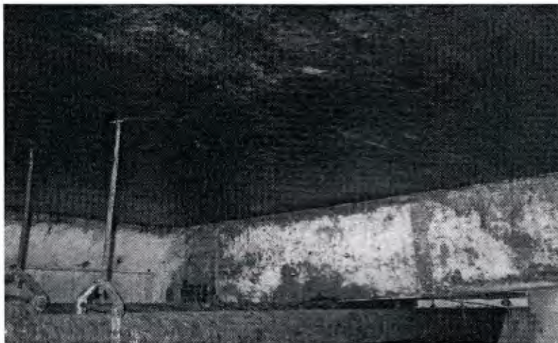
Figure 8. Finished installation of graphite laminate on the south side lane.
