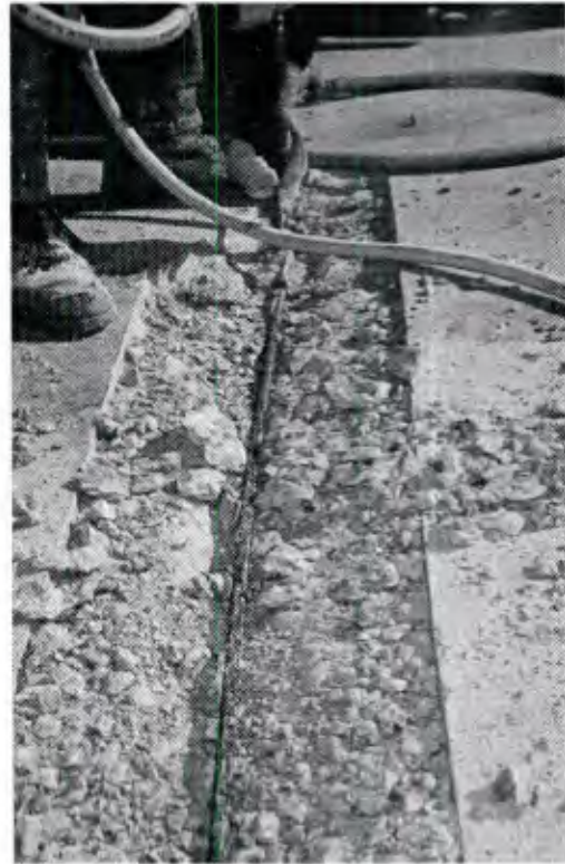
Figure 23. Removing deteriorated concrete with small pneumatic hammer.
