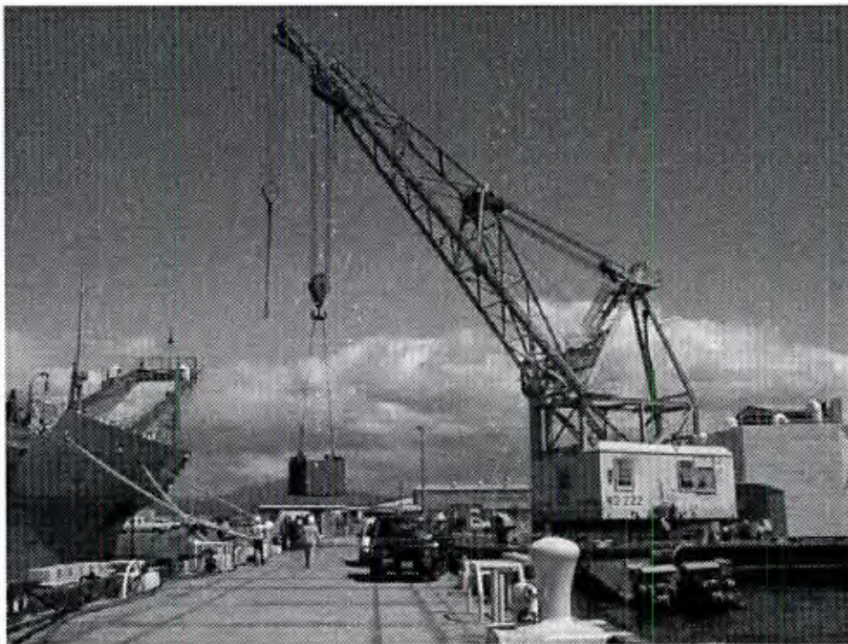
Figure 45. Applying calibrated weights to the deck for proof loading upgrade areas.
