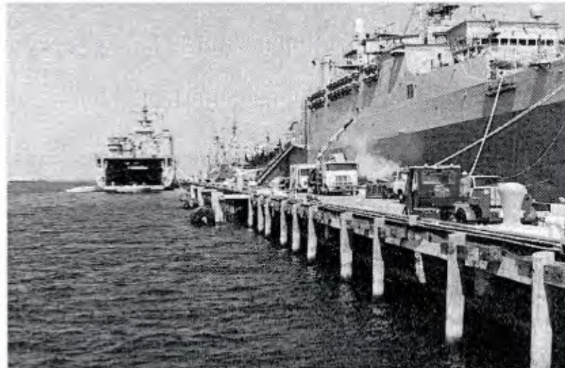
Figure 1. Pier 12 San Diego Naval Station
