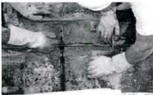
Figure 24. Hand packing concrete repair material.
