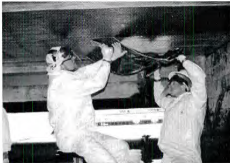
Figure 39. Hand application of in situ impregnated laminate sheet.
