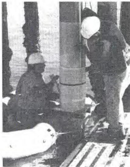
Figure B38. Installing pile confinement upgrade demonstration on AWTTS pile.
