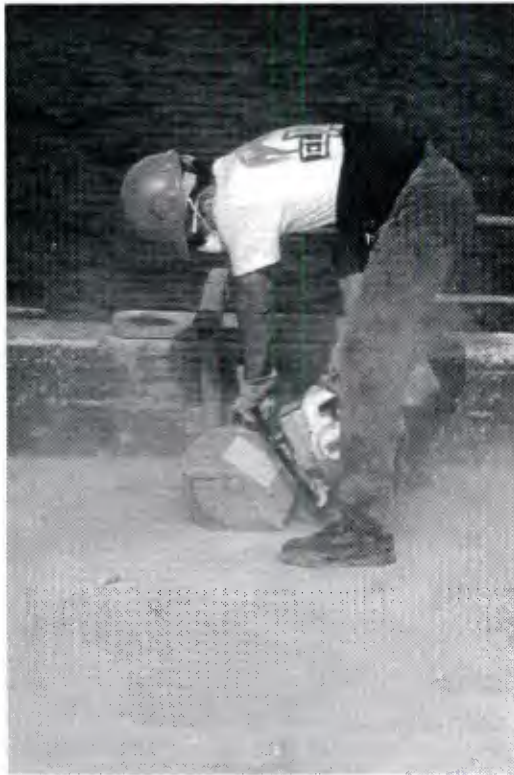
Figure 22. Saw cutting perimeter of concrete repair area.
