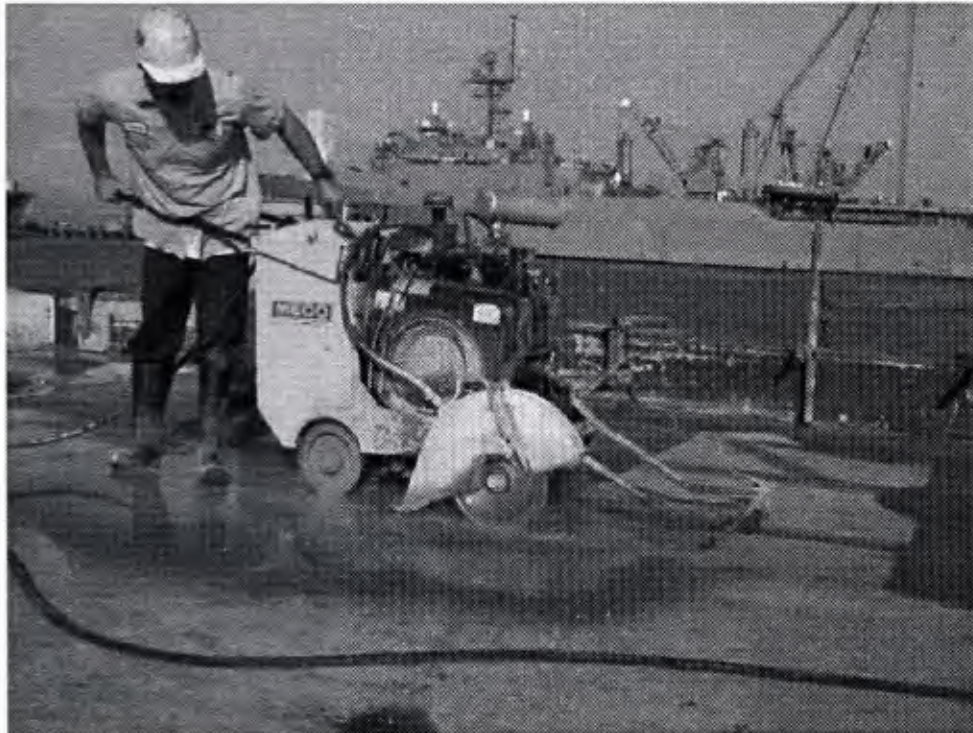
Figure 30. Saw cutting slots on deck surface.
