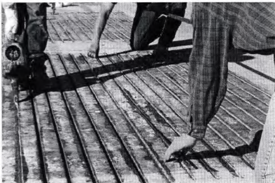
Figure 31. Embedded high strength carbon rod in top of deck over pilecap.
