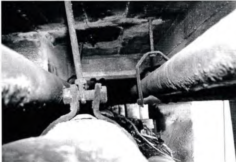
Figure 15. Utility hangers anchored to Pier 12 deck.
