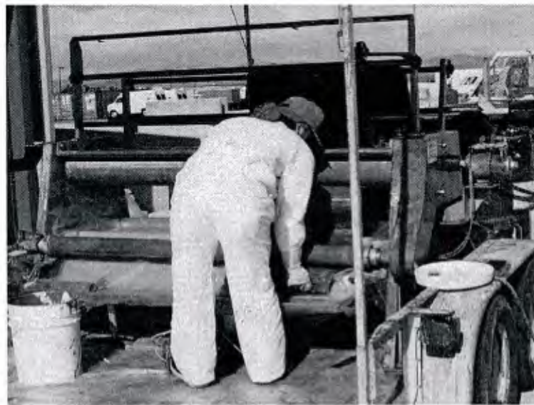
Figure 38. Saturator for in situ epoxy impregnation.
