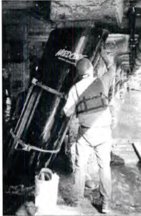
Figure 41. Placing cylindrical composite shell around pile.
