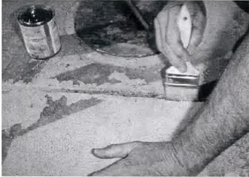
Figure 19. Applying polyurethane primer to construction joint crack.
