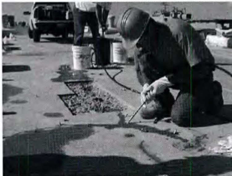
Figure 18. Injecting polyurethane into cracks on deck surface.
