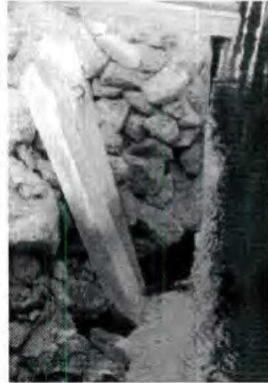
Figure 1. Piles in the harbor
