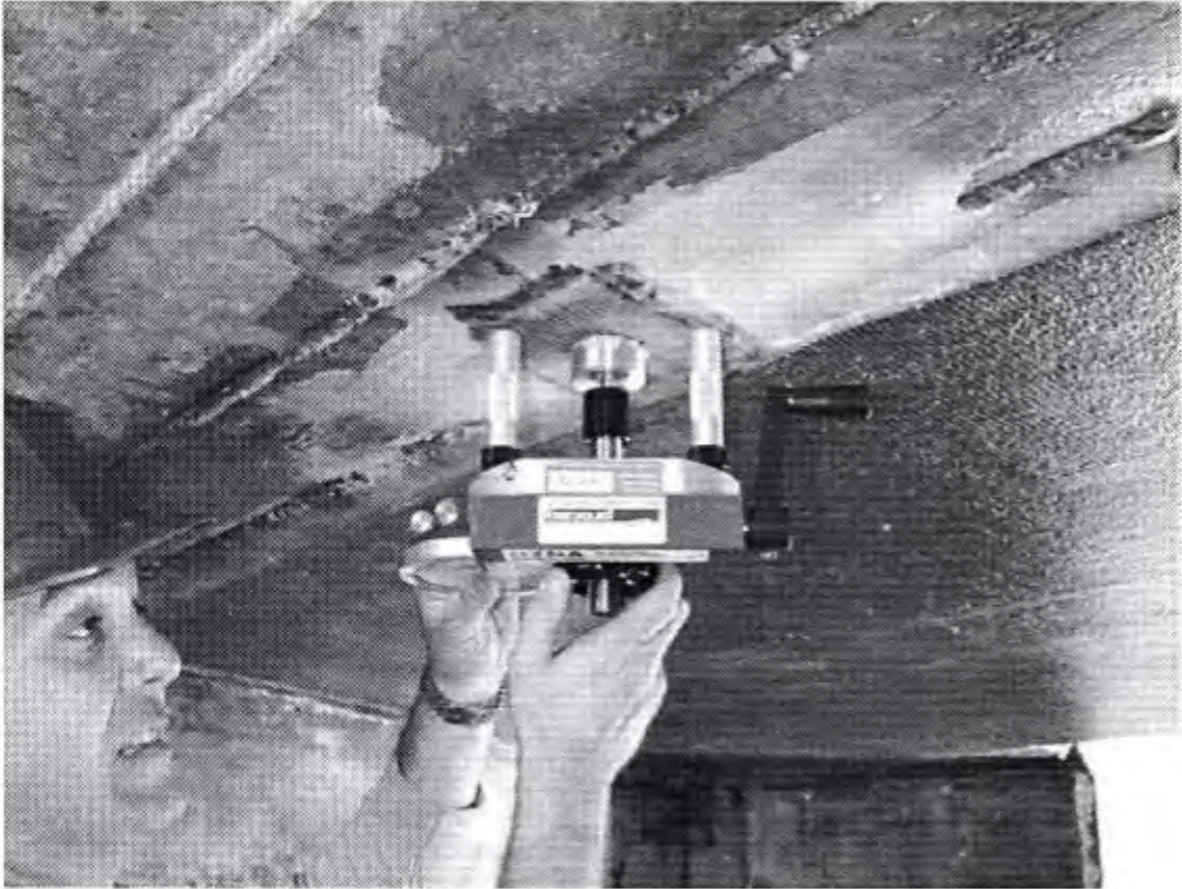
Figure B43. Bond testing with pull-off tester.
