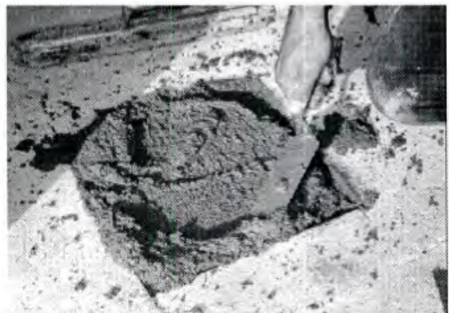
Figure 25. Concrete repair with small hand tools.
