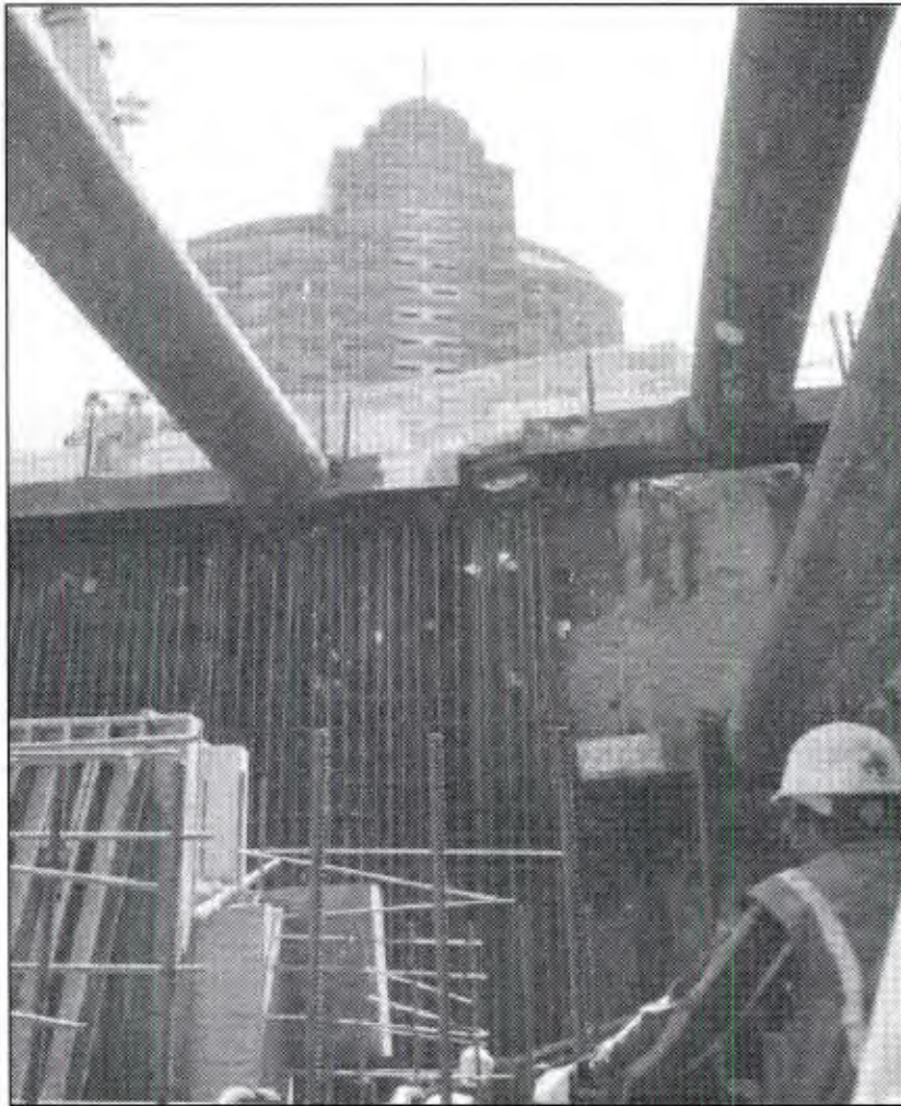
Construction of Muni-Metro Turn Back, San Francisco, California
