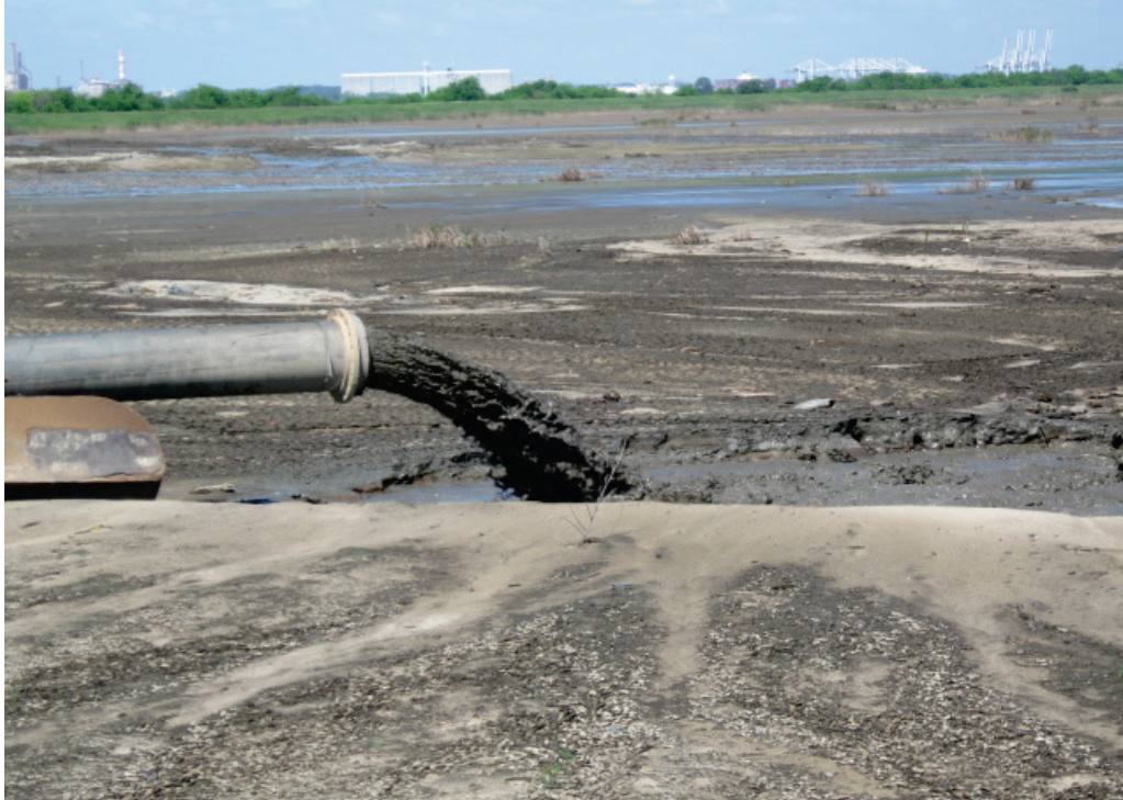
Figure 3. A view of one Dredged Material Containment Area receiving dredged material in the Savannah Harbor Navigation Project, Savannah Harbor, USACE Savannah District, GA. The material deposited in this area was later repositioned to create bird habitat.
