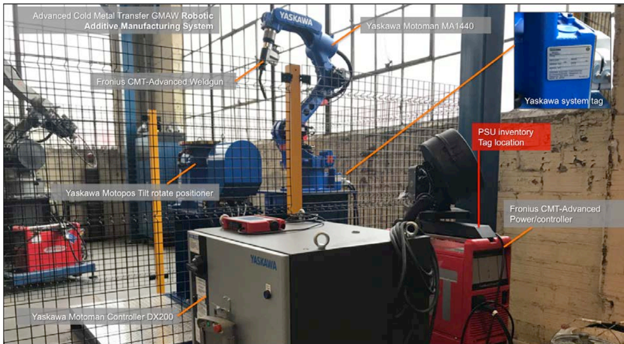
Figure 5. Completed system set-up after installation and test run.
