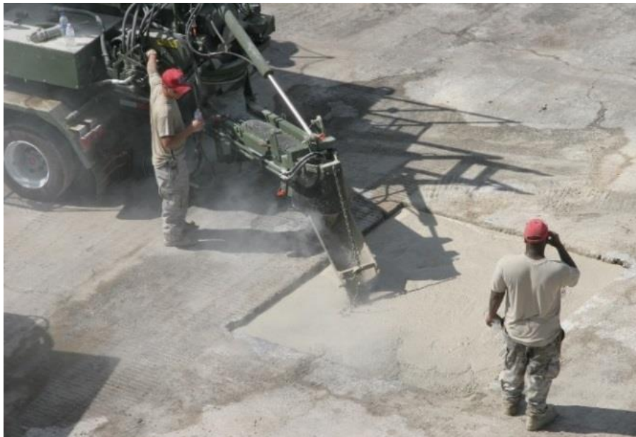
Figure 1. Rapid-setting flowable fill wet placement method.
