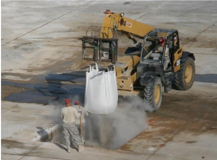
Figure 2. Rapid-setting flowable fill dry placement method.
