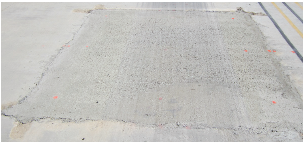
Figure 20. Repair 2, overall, 112 passes.
