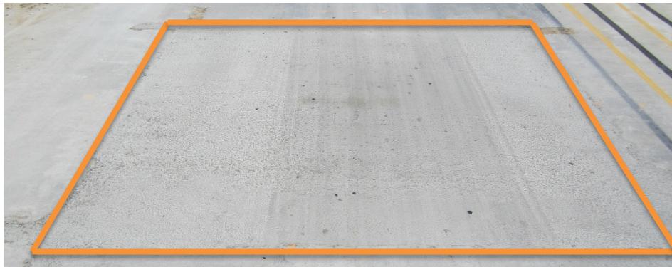
Figure 33. Repair 4, overall, 112 passes.
