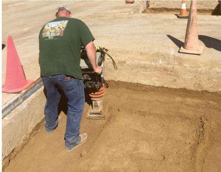
Figure 7. Compaction of brown CL clay subgrade.
