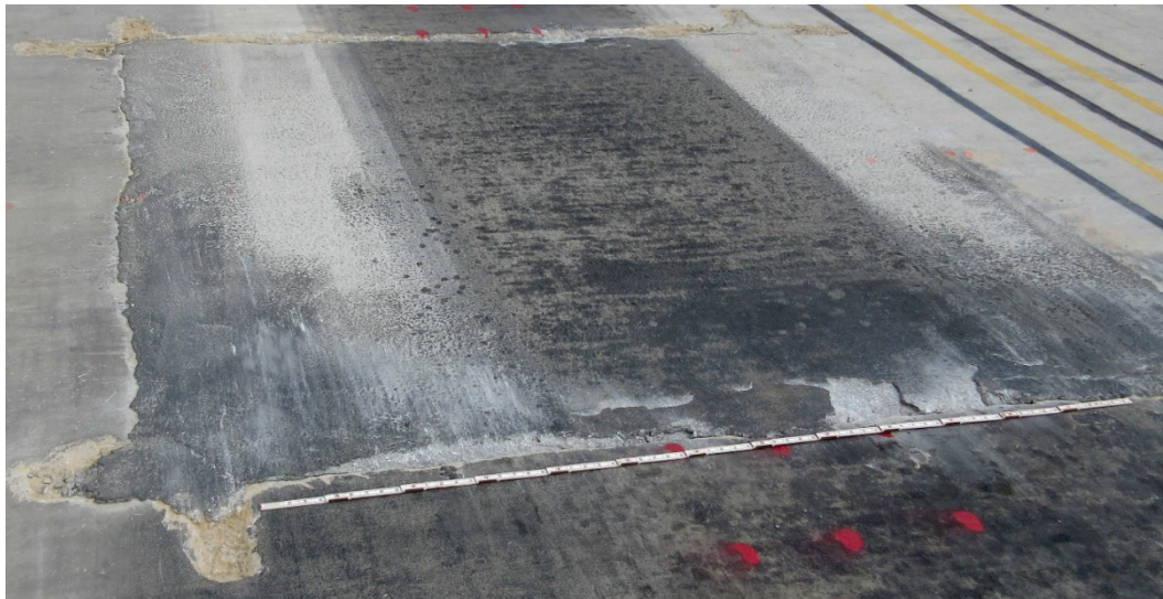
Figure 29. Repair 2, overall, 2,000 passes.
