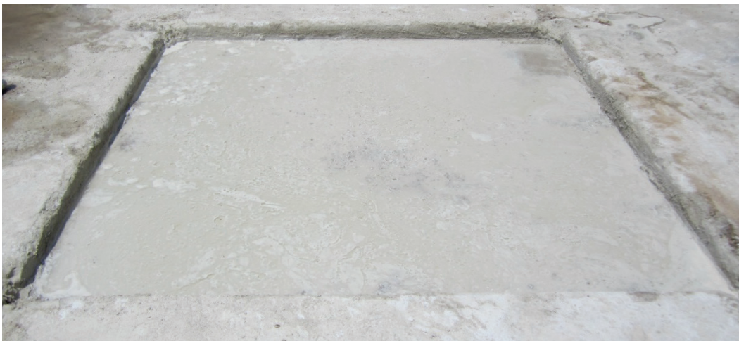
Figure 12. Completed rapid-setting flowable fill placement after 30 min of cure time.
