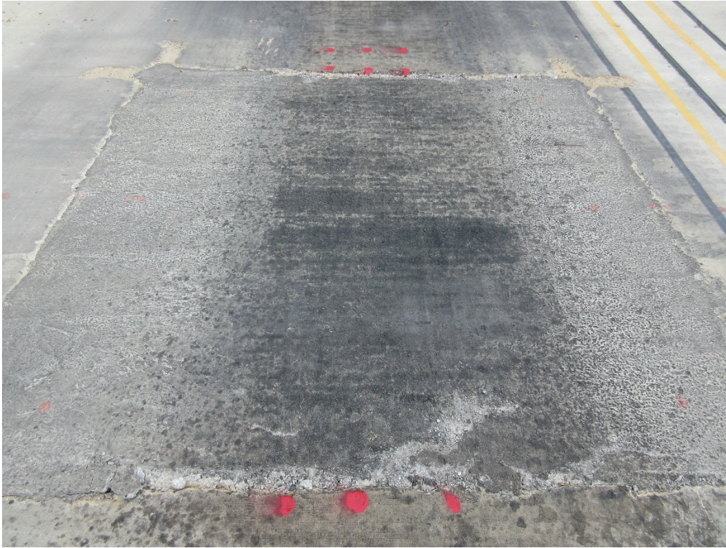
Figure 26. Repair 1, overall, 2,000 passes.
