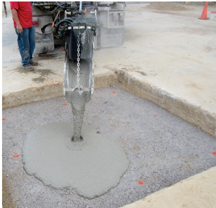
Figure 13 . Placement of rapid-setting concrete capping material.
