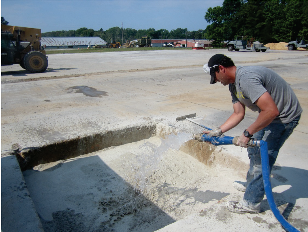
Figure 11. Metering of water over dry rapid-setting flowable fill.
