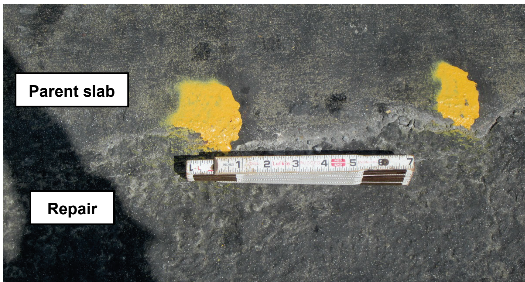
Figure 35. Repair 4, rear edge, 2,000 passes.
