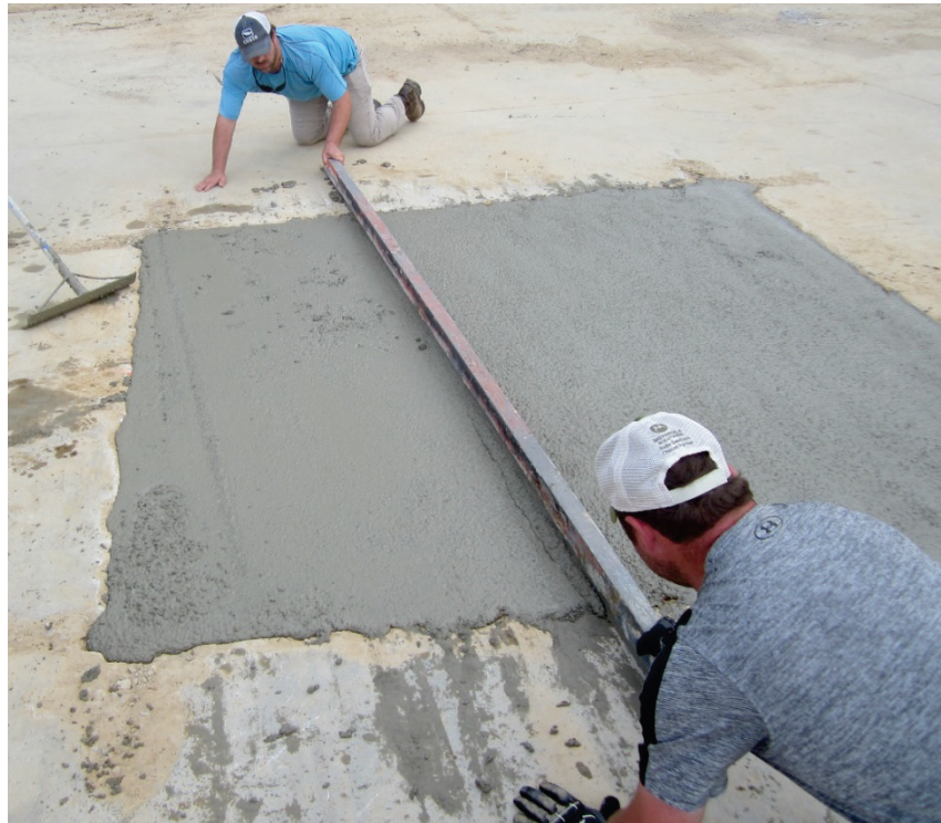
Figure 14. Screeding of rapid-setting concrete capping material.
