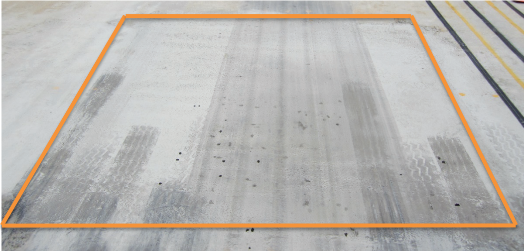
Figure 34. Repair 5, overall, 112 passes.
