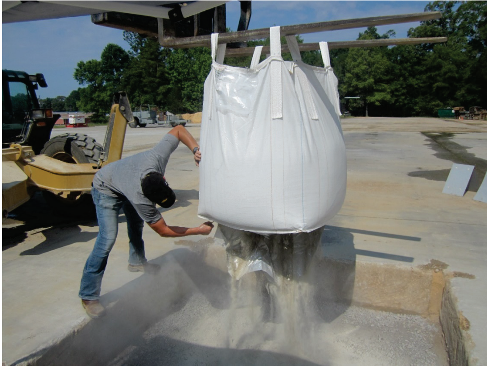
Figure 9. Placement of rapid-setting flowable fill material.
