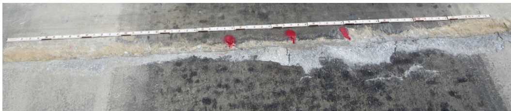
Figure 30. Repair 2, rear edge, 2,000 passes.
