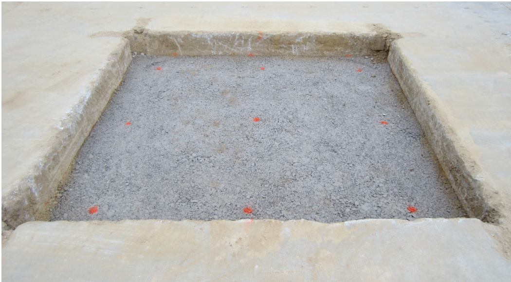
Figure 8. Compacted crushed stone backfill material.
