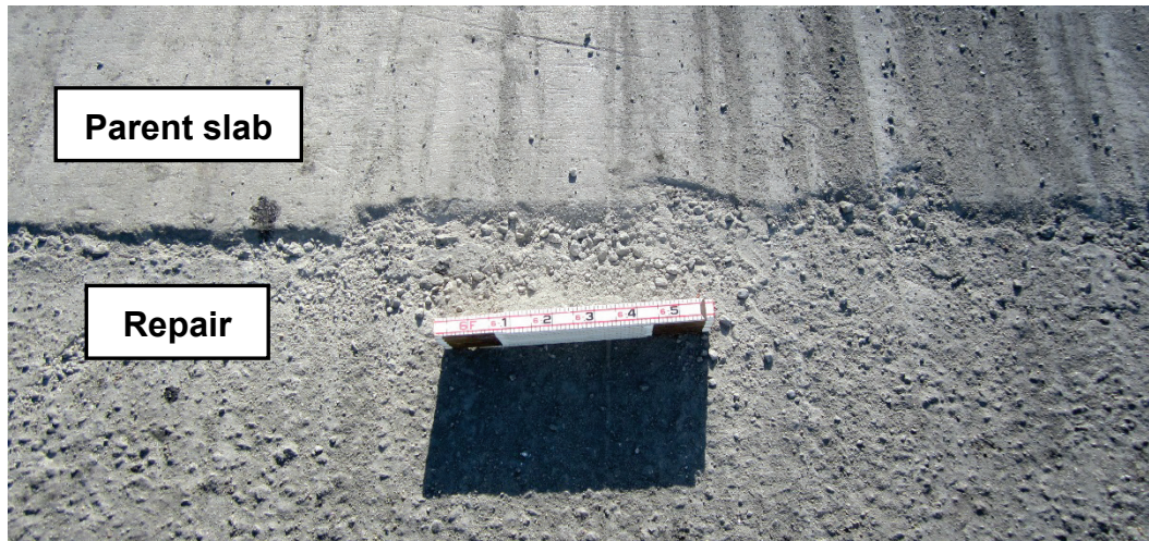
Figure 23. Repair 1, rear edge deterioration, 1,000 passes.
