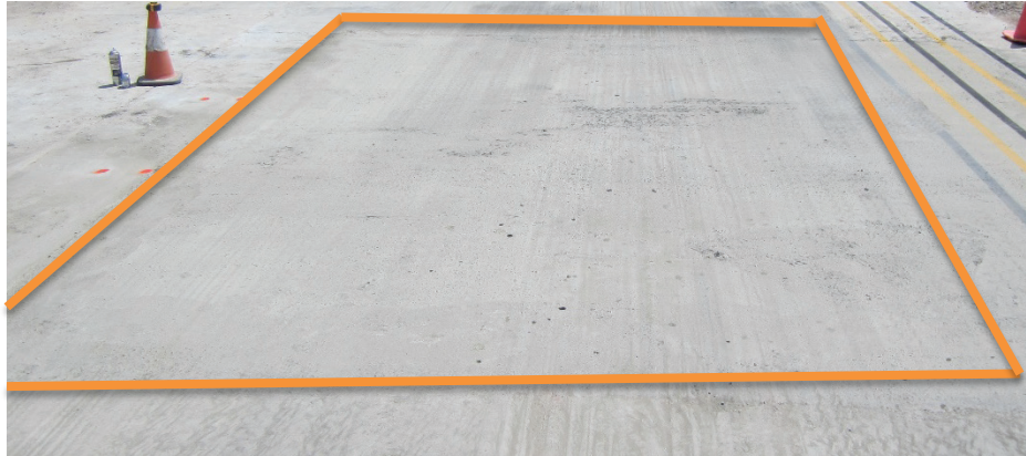
Figure 21. Repair 3, overall, 112 passes.
