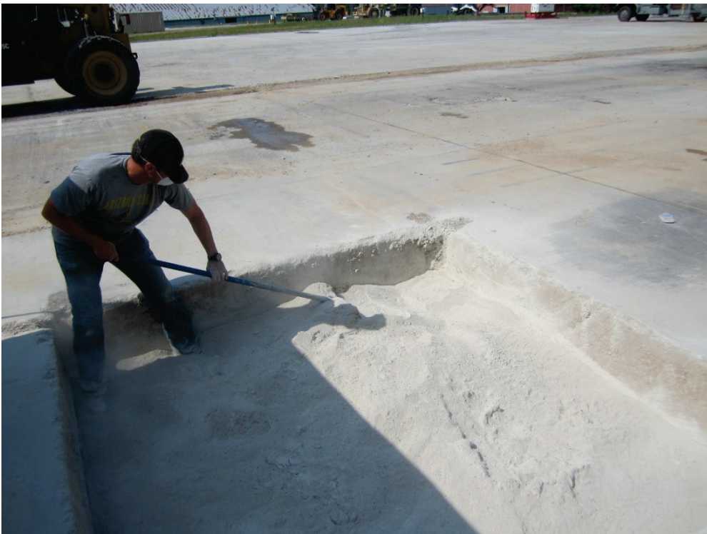
Figure 10. Leveling of dry rapid-setting flowable fill material.
