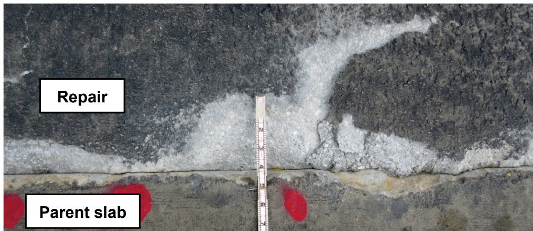
Figure 27. Repair 1, front edge, 2,000 passes.
