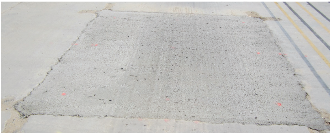
Figure 19. Repair 1, overall, 112 passes.
