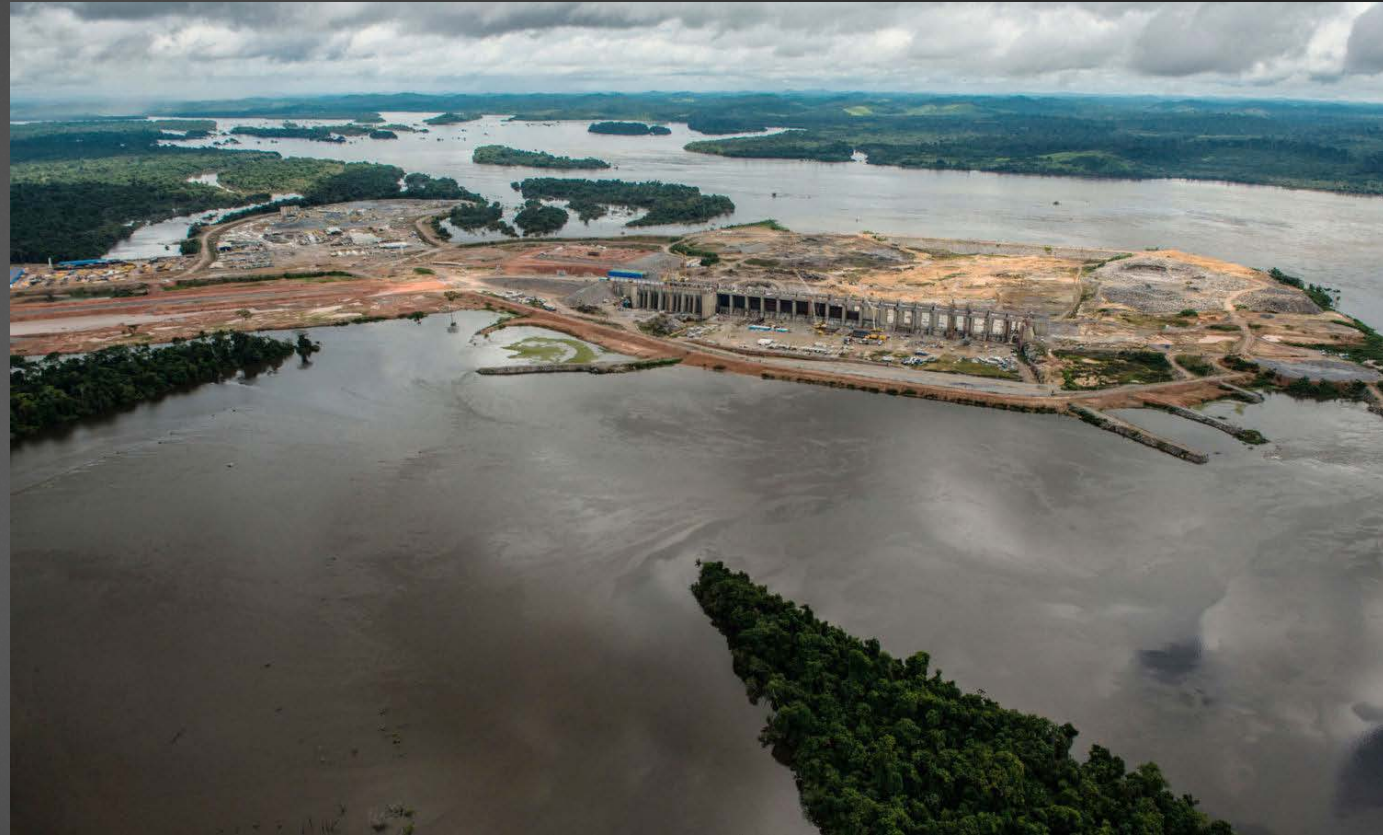
Belo Monte Mega-Dam under construction
