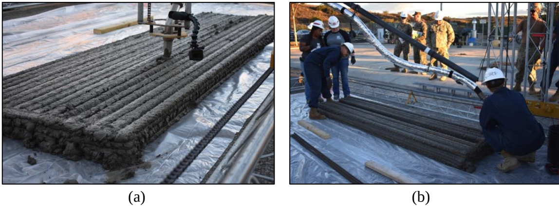
Figure 11. (a) Printing beam 1; (b) placing rebar on beam 1.
