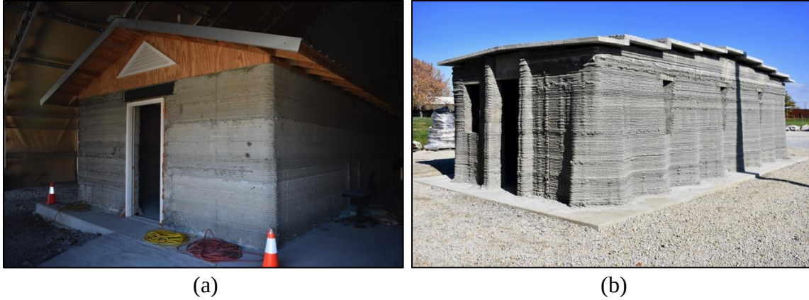
Figure 8. (a) B-Hut 1, a 48m 2 building printed in stages over the span of several weeks. (b) B-Hut 2, a 48m 2 chevron-style building printed in 14 hours over the span of five days.
