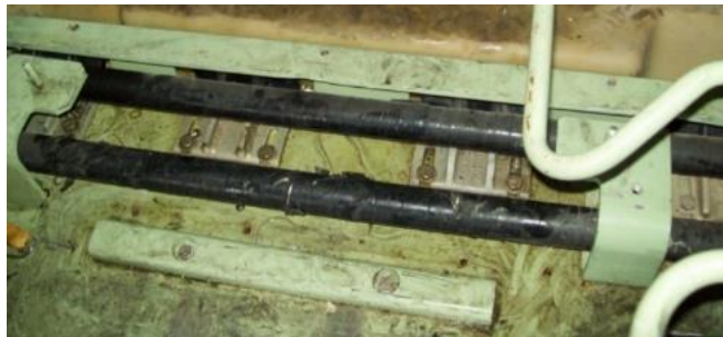
Fig. 5 Taped bars damaged during vehicle assembly
