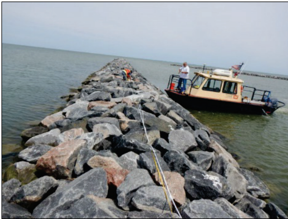
Figure 5. Crew setting up transects for future analysis of structural stability.
