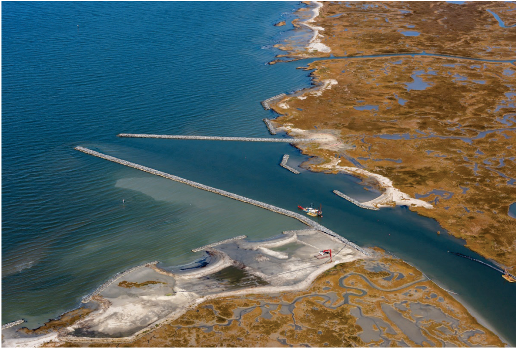
Figure 2. Aerial view of the completed jetties and sill at the Rhodes Point Navigation Project in June 2018, prior to dredging of the channel (photo credit: Coastal Design & Construction, Inc).
