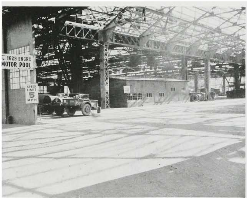
Entrance to Motor Pool (Japan)
