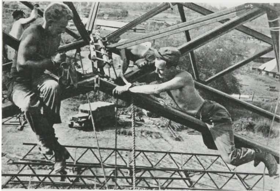
Riggers at work on hangar
