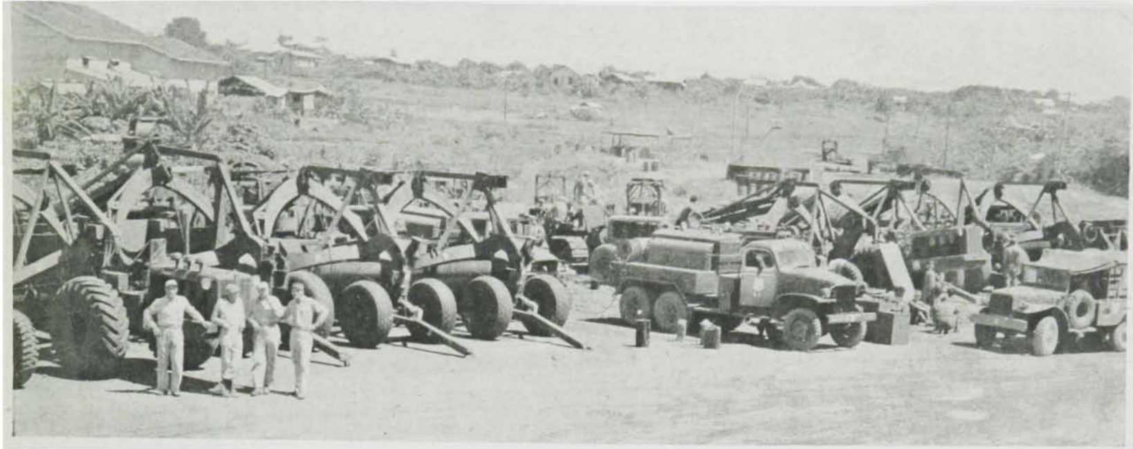
Section of Heavy Equipment area, Quezon City, Philippines
