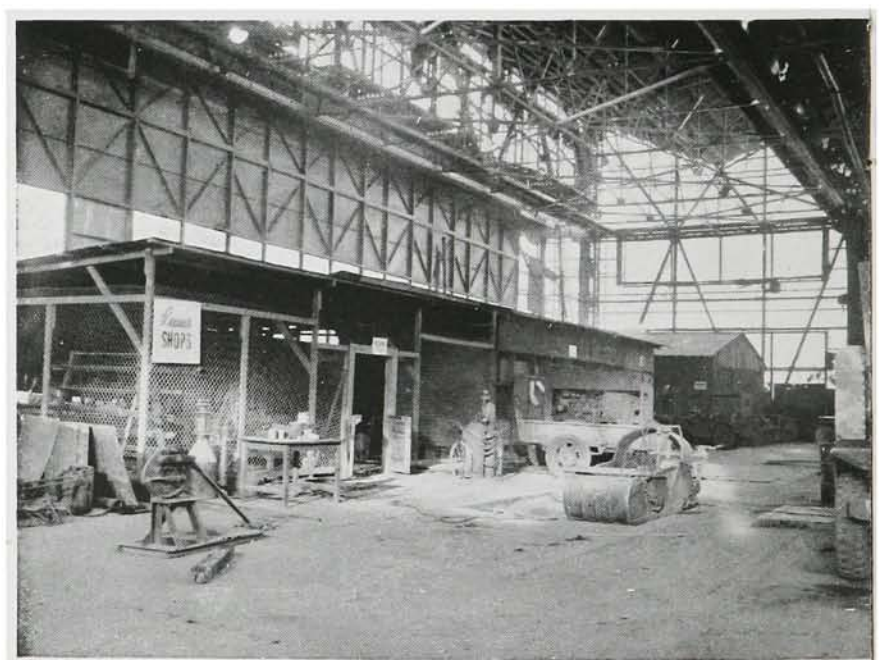
Repair section, motor pool (Japan)
