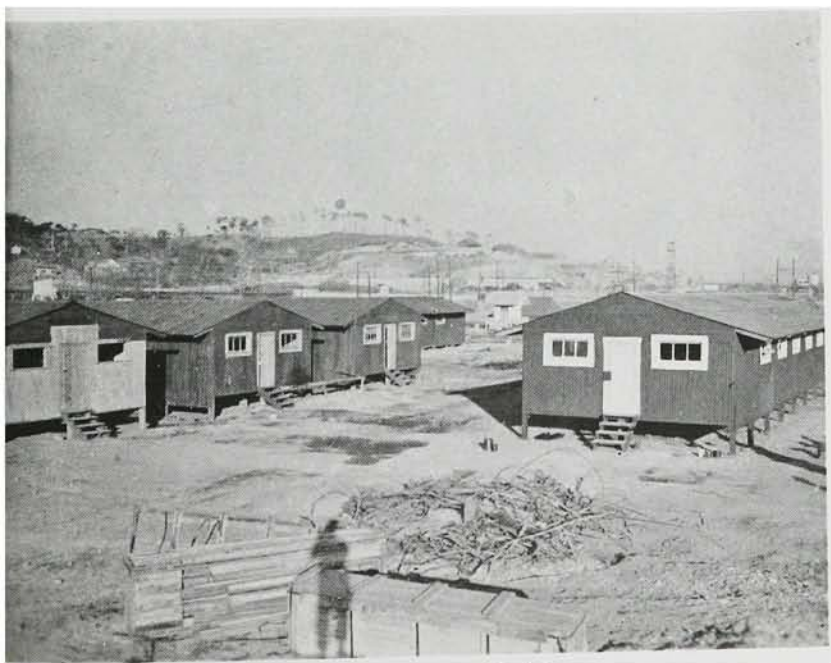
Military stockade project, Yokohama
