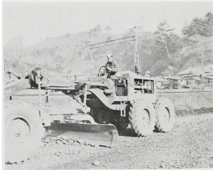
Grading the Yokosuka Road (Japan)
