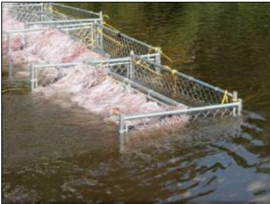
Figure 1. Gabion basket with snare booms in the Kalamazoo River during cleanup efforts. (Dollhopf and Kimble, 2016)
