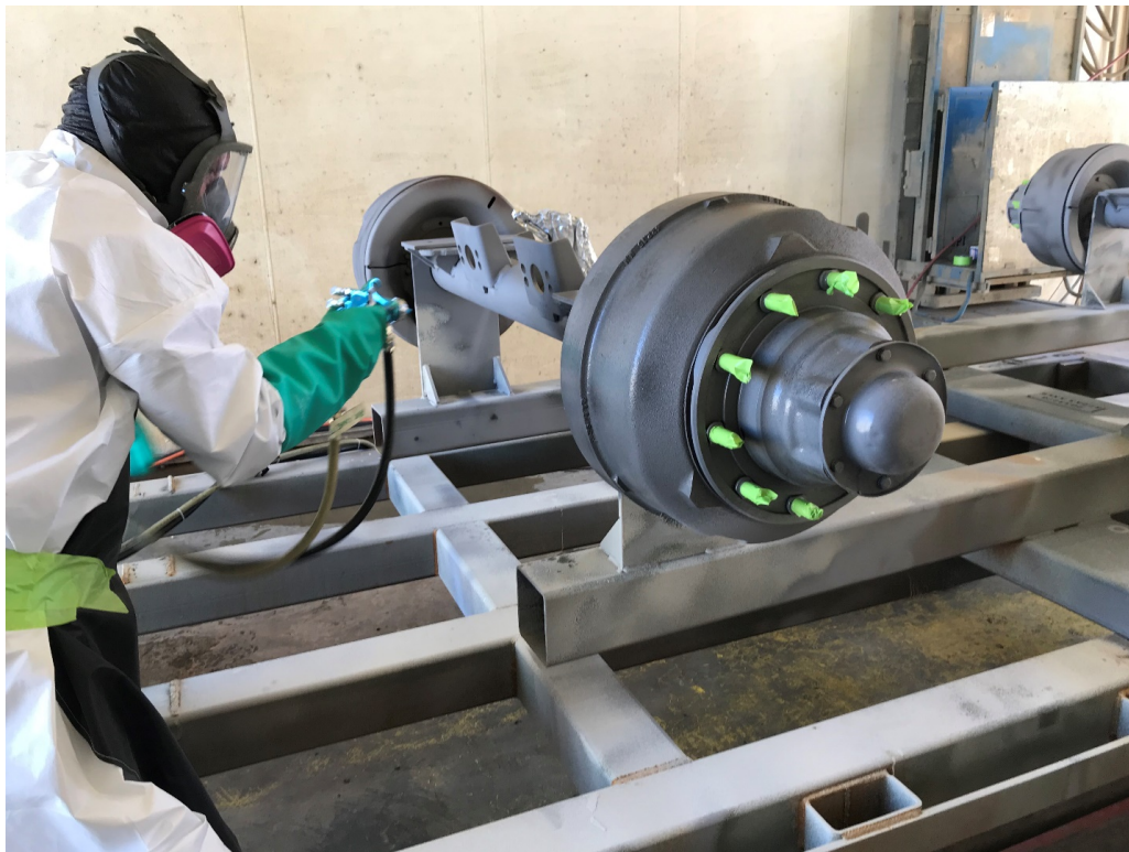
Fig. 4 Axle assemblies being sprayed with Bonderite M-NT 7400
